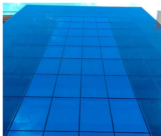
Fig. 4.2 a-Si BIPV glazed facade. Source: Onyx Solar.
