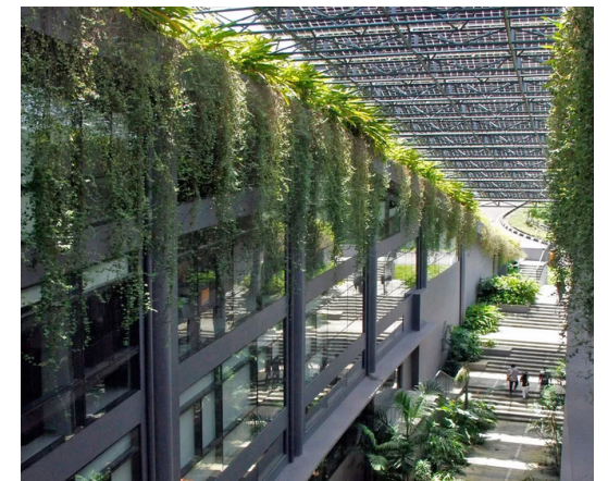
Fig. 4.15 Canopy, interior view. Source: Stapati.
