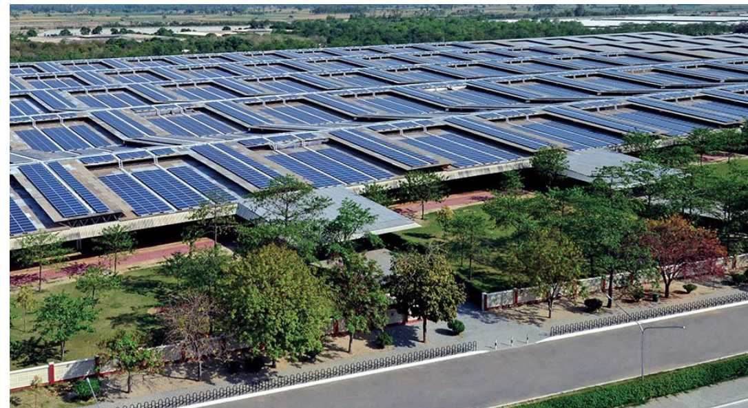
Fig. 1.12 RSSB-EES in Beas. Source: L&T Construction.
