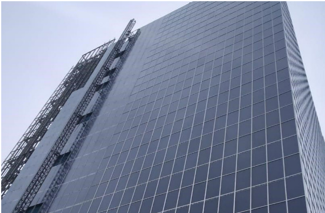
Fig. 1.13 CTRLS Data Center, Mumbai. Source: U-Solar.
