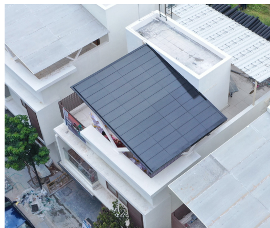
Fig. 4.7 . Aerial view of the PowerRoof. Source: SunEdison
