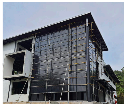
Fig. 4.11 Curtain wall under construction. Source: TopSun
