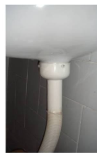
Fixing of Membrane Valve at urinal pot
