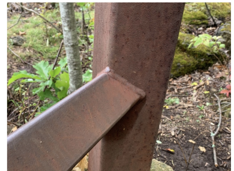
Figure 2: Square HSS Diamond-Bird-Beak (DBB) T-connection example
