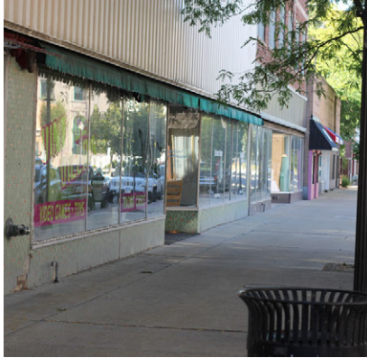
The Former Sears Building
