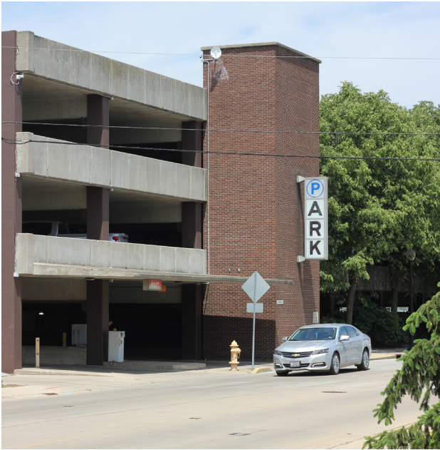
Restriping crosswalks and adding curb extensions would complement the rehabilitation efforts planned for the parking garage.
