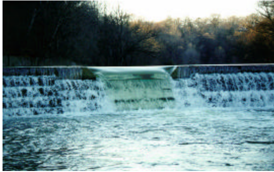
Old Mill Dam Notching, Toronto
