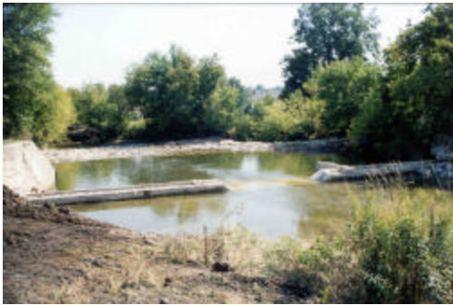
McFall Dam Notching and Rocky Ramp, Bolton
