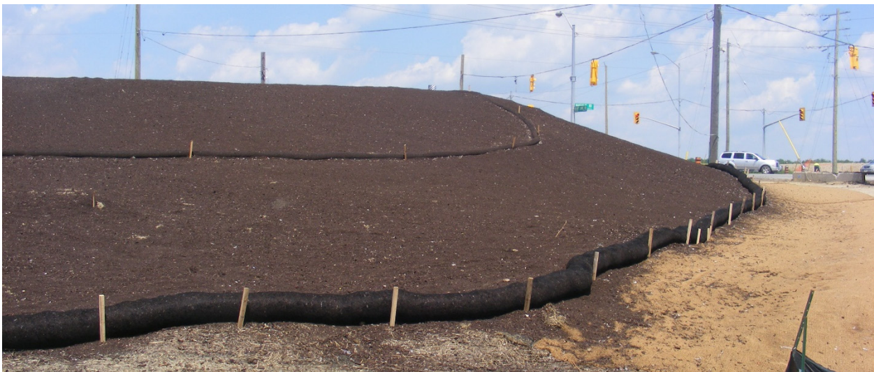
Figure B2-6: Filter socks installed along contours of a slope
