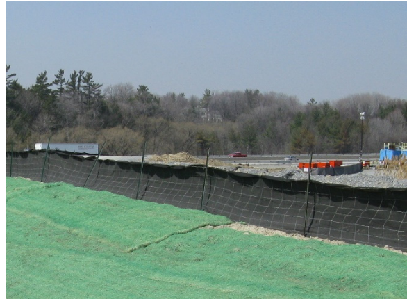
Figure B2-1: Sediment control fence
