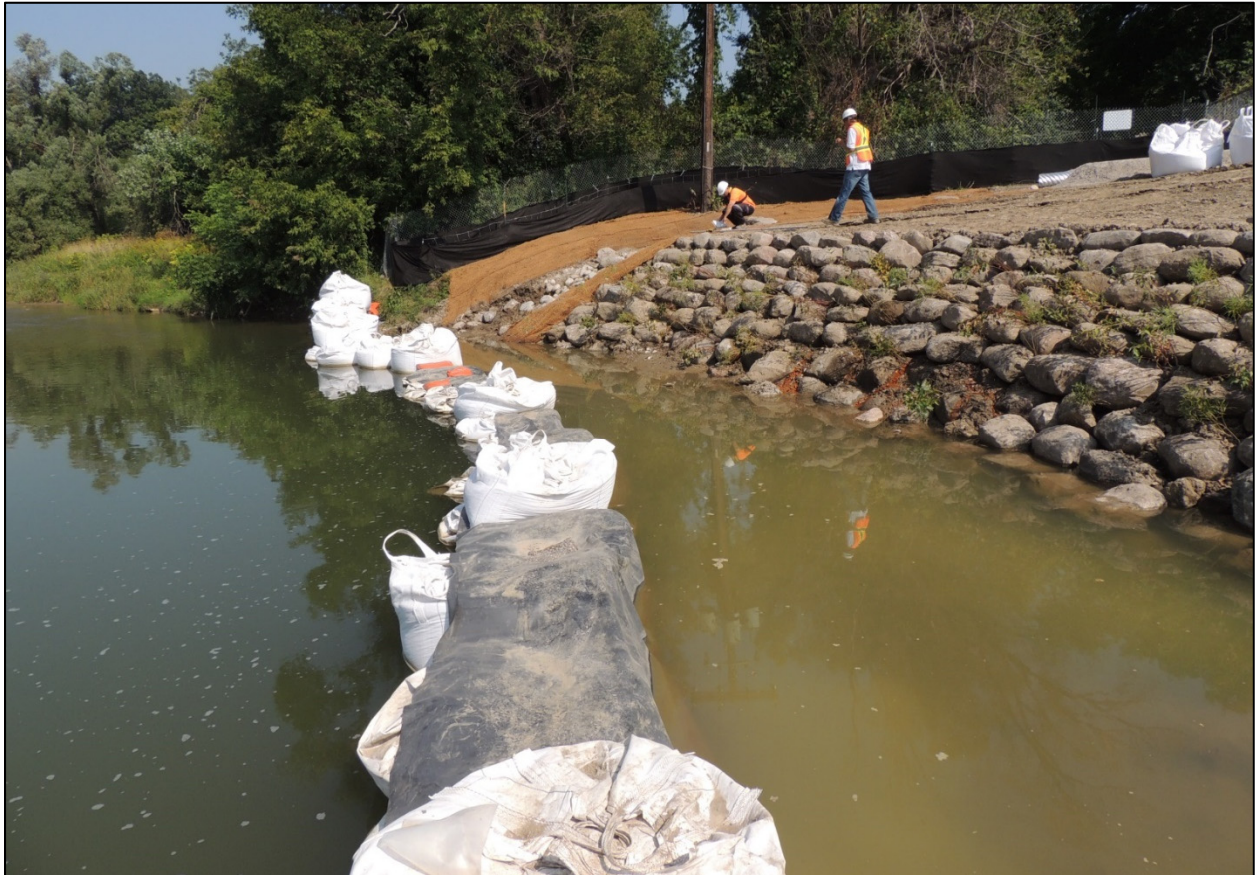
Figure C5: Waterproof isolation barrier (cofferdam)
