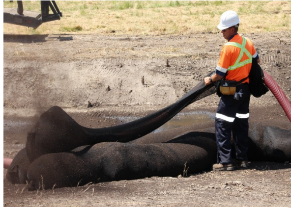
Figure B2-4: Filter sock being filled on site
