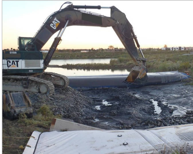
Figure 7.14: In-water worksite isolation
