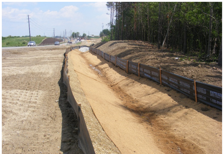
Figure B1-4: Stabilized interceptor swale
