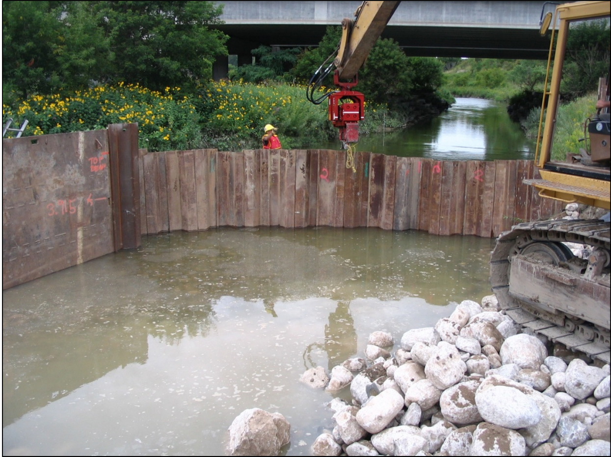
Figure C13: Sheet pile isolation wall
