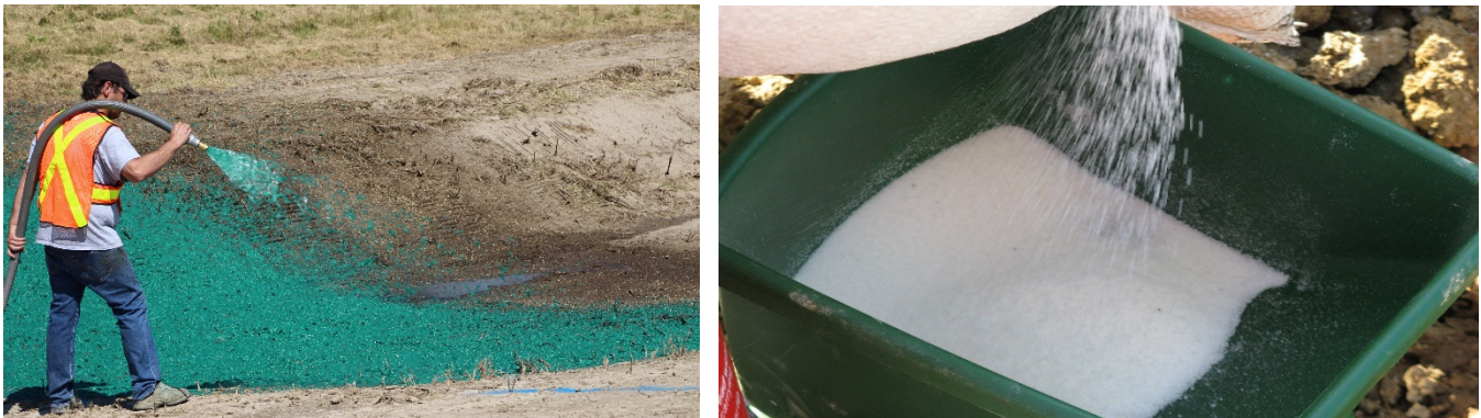
Figure B1-17: Application of hydroseed containing tackifier (left) and granular anionic polyacrylamide (right)
