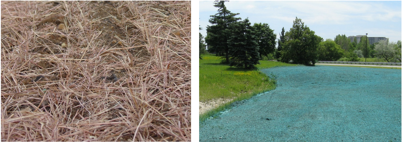
Figure B1-7: Dry straw crimped into place (left) and hydromulched area (right)
