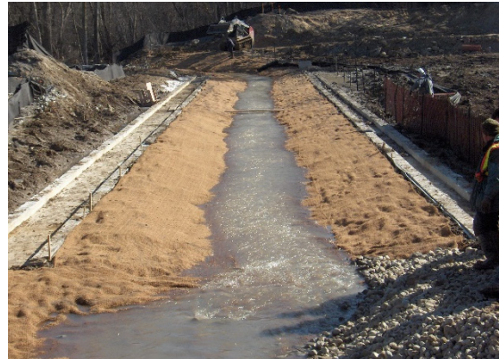
Figure 9.1: Watercourse diversion during construction is exempt from requiring a PTTW.
