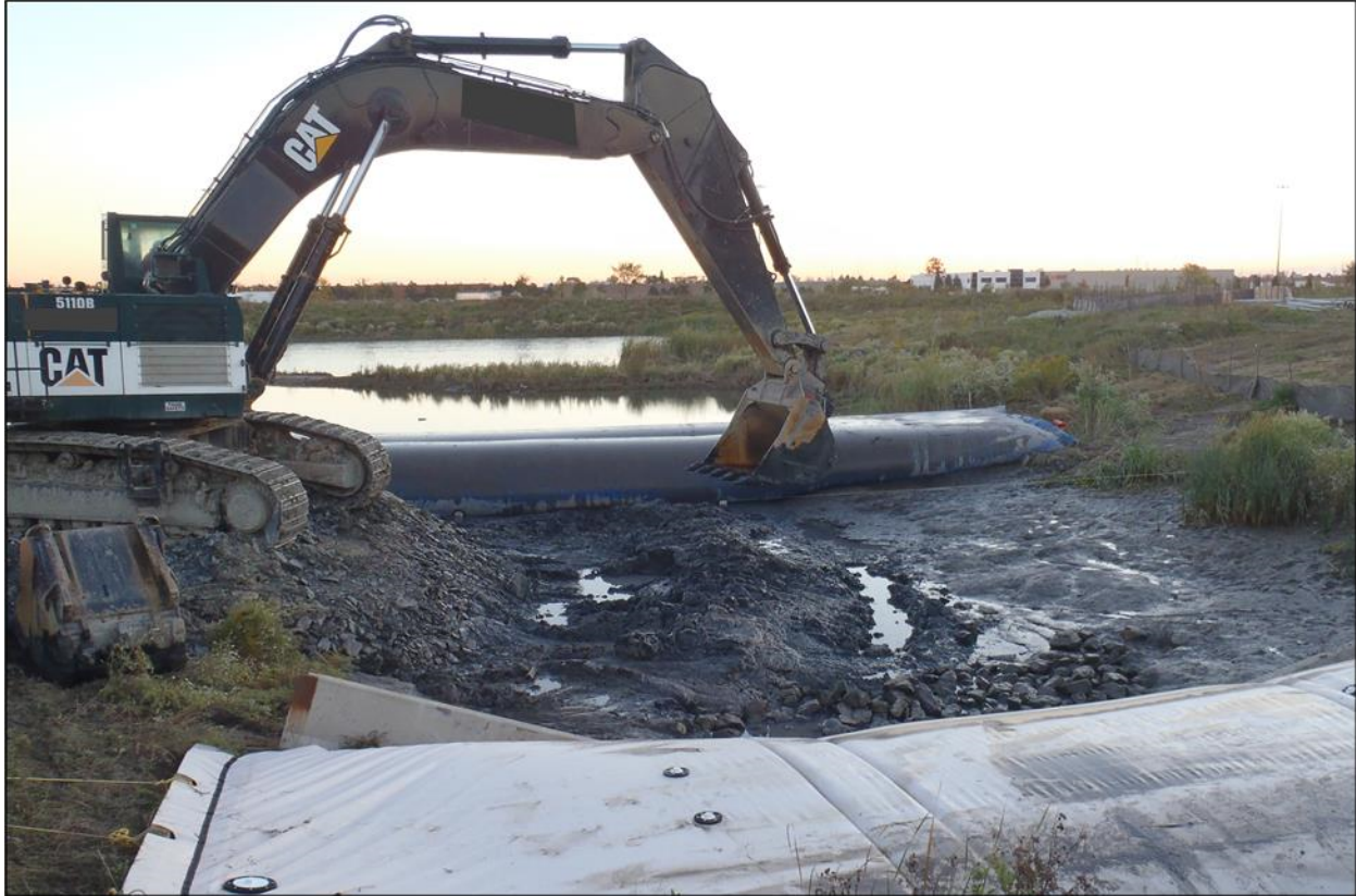
Figure C14: Work area isolation using water-filled bladders
