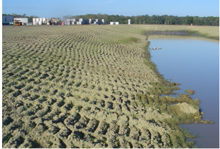
Figure B1-6: Track walking applied to bare soil
