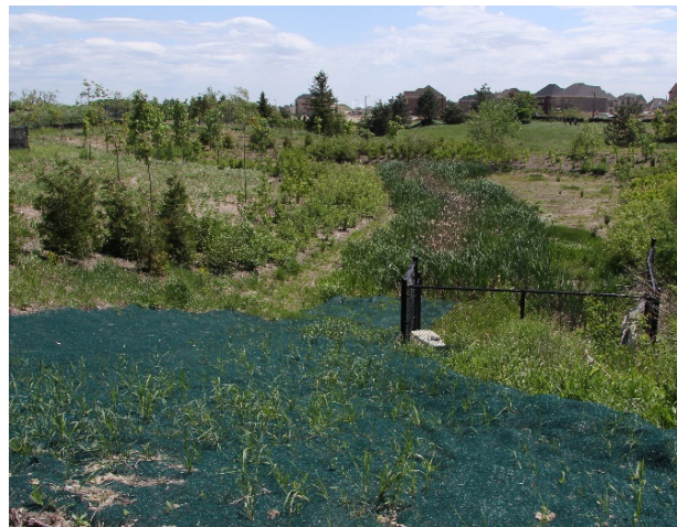
Figure 7.7: Soil stabilization with a rolled erosion control product
