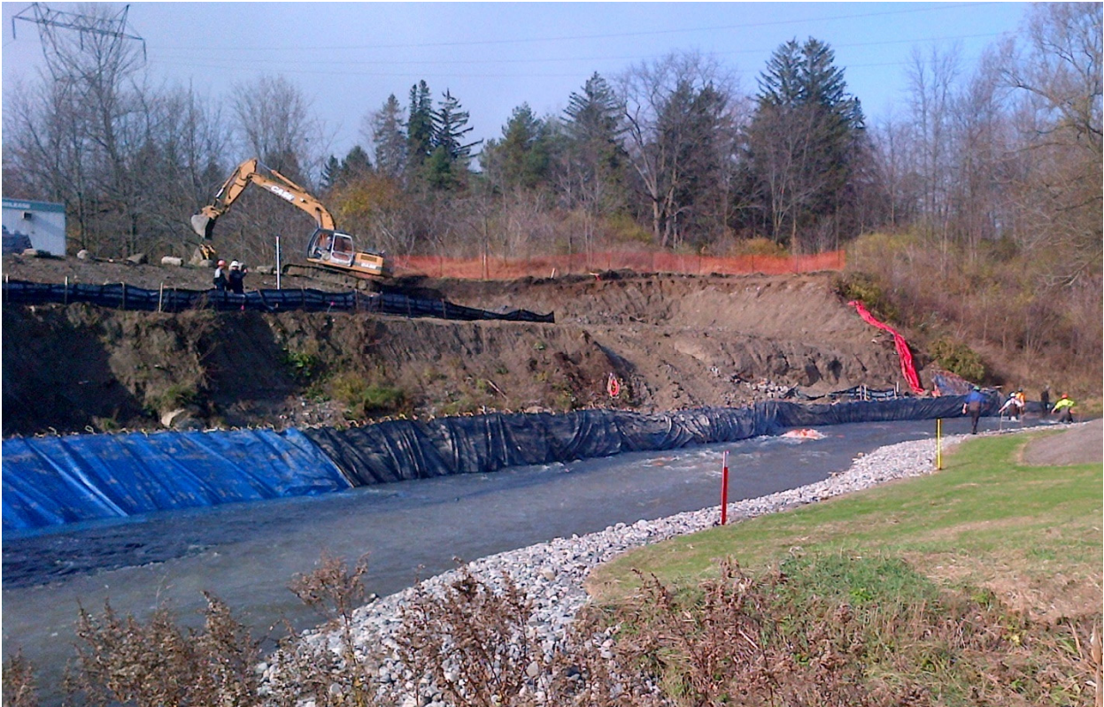
Figure C15: Work area isolation with a portable dam system
