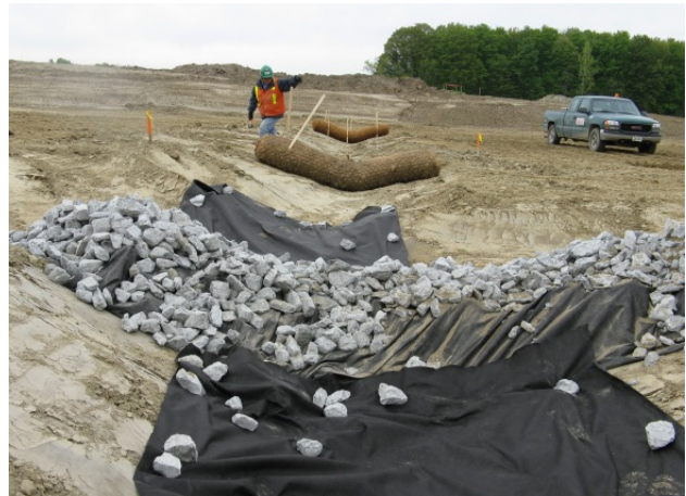
Figure 10.7: Maintenance of rock check dams
