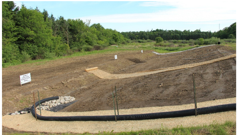
Figure B1-3: Slope drain
