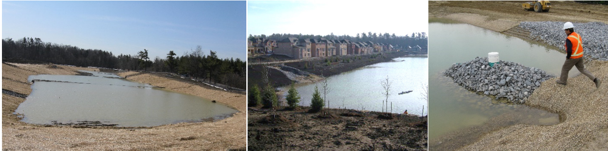
Figure B2-19: Sediment control ponds
