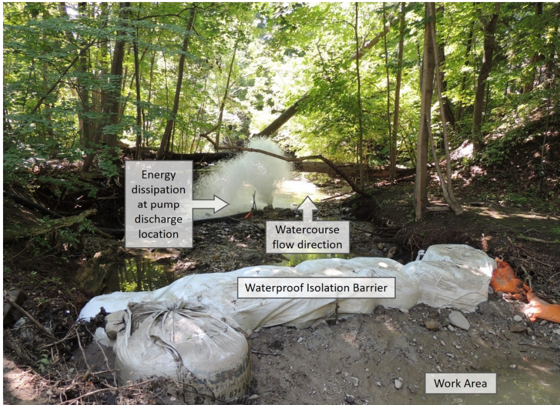
Figure C11: Energy dissipation at pump discharge location during bypass pumping
