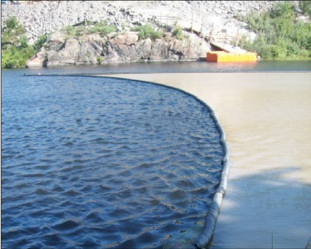
Figure C2: Sediment curtain installed in a lake
