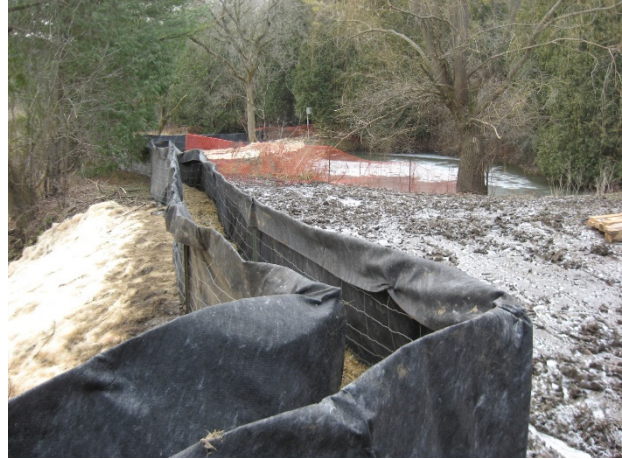
Figure B2-2: Double row sediment control fencing
