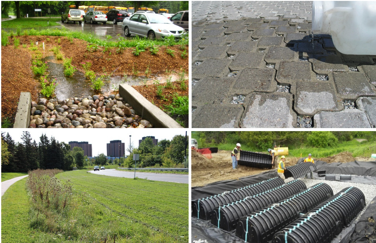
Figure 7.16: Infiltration LID practices that can be vulnerable to impacts from construction. Clockwise from top left – bioretention area, permeable interlocking concrete pavement, underground infiltration chambers, enhanced grassed swale.
