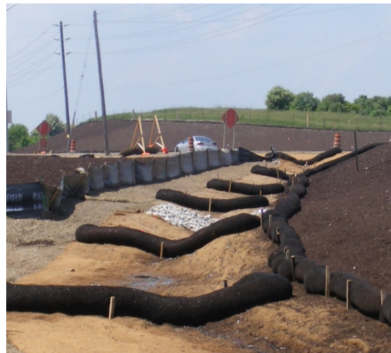
Figure 4.6: Erosion control blanket (left) and filter socks applied as sediment control check dams (right).
