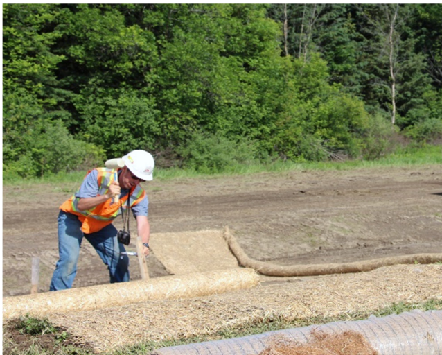
Figure 4.6: Erosion control blanket (left) and filter socks applied as sediment control check dams (right).
