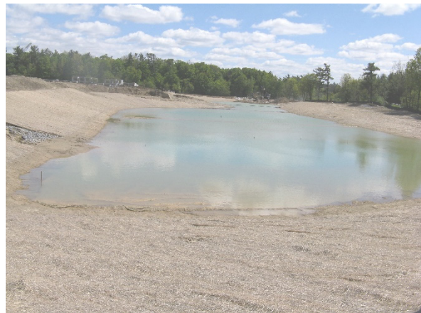
Figure 7.8: Temporary sediment control pond
