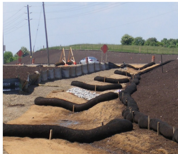
Figure B2-7: Filter socks installed in a swale
