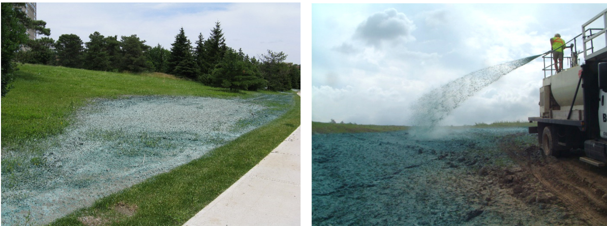
Figure B1-10: Hydroseeded area (left) and application of hydroseeding (right)
