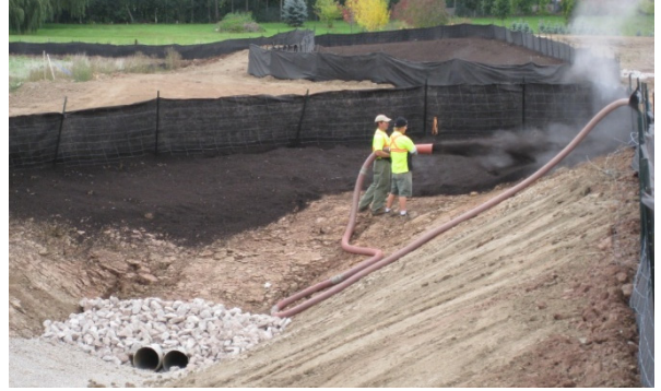
Figure B1-11: Pneumatic seeding with growing media
