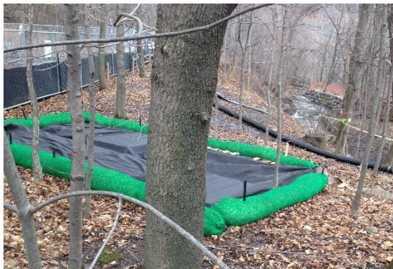
Figure 7.10: A multi-barrier/treatment train approach to dewatering with a sediment bag
