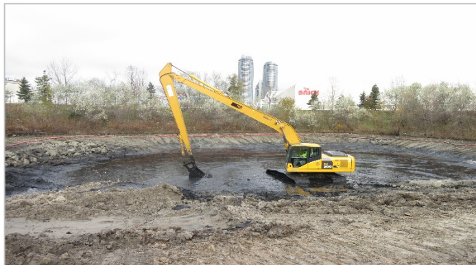
Figure B2-20: Sediment removal from a pond
