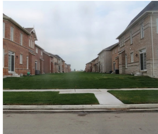
Figure 7.6: Subdivision after final stabilization
