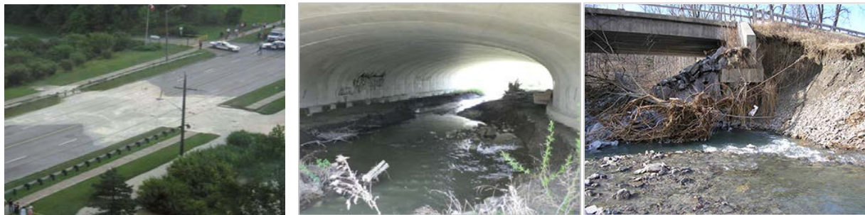
Figure 2: Impacts of crossing infrastructure on natural hazards (a) impacts on flooding, (b) impacts on channel migration, and (c) impacts on erosion
