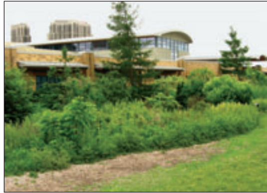
Humberwood Community Centre in Toronto features many green building attributes including naturalized landscaping, stormwater bioretention areas and porous paving. Photography by Dean Young
