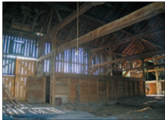
Inside the McVean Barn
