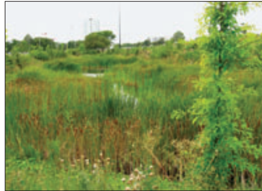
Retrofitted stormwater management pond near Colborne Lodge Drive in Toronto. Photography by Dean Young
