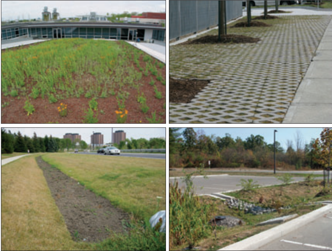
From top left: green roof, porous pavement, grassed swale, parking lot bioretention area
