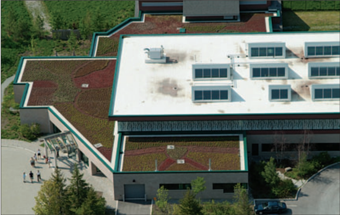
The Earth Rangers building at the Living City Campus at Kortright is a certified green building. Photography by Rose Hasner
