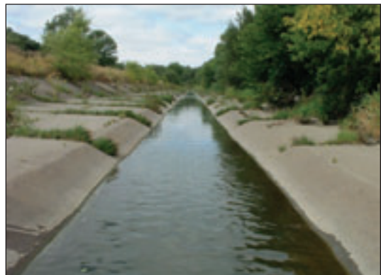
Portions of Black Creek have been channelized to reduce risk of flooding. Photography by Jamie Duncan
