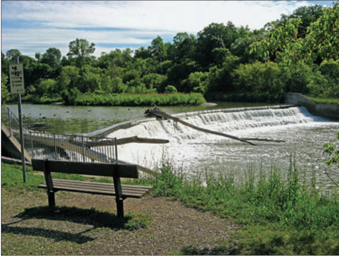
Weir on the main channel of the Humber River that is a high priority for modification to improve fish passage. Photography by Dean Young
