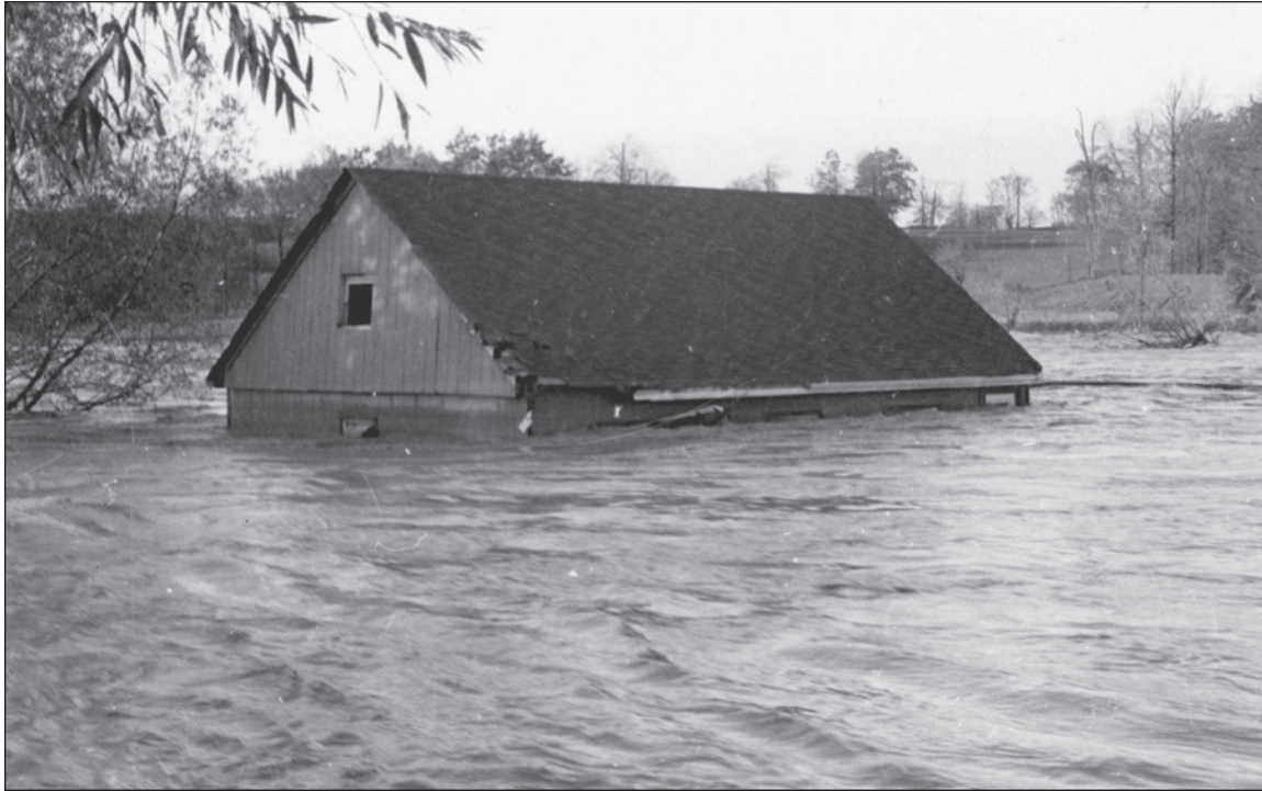
Home flooded following Hurricane Hazel, the largest storm event on record in the watershed.
