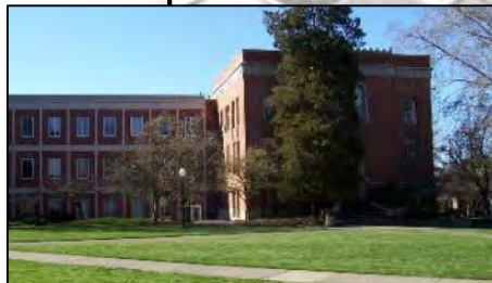
Condon Hall Deferred Maint.
