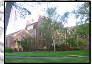
Hendricks Hall Deferred Maint.
