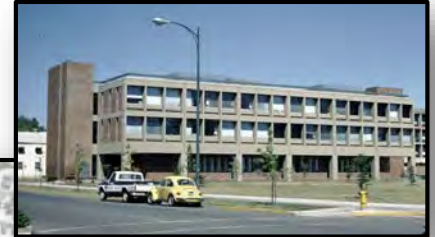
Huestis Hall Deferred Maint.
