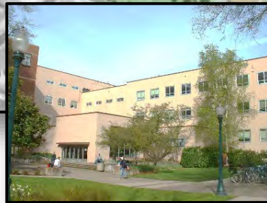
Pacific Hall Phase 2 Classroom 123 & Lobby
