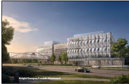
Knight Campus Phase 3 Research Building
