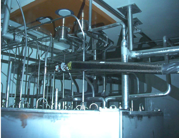
Fig. 21- Inspection of a pipe
