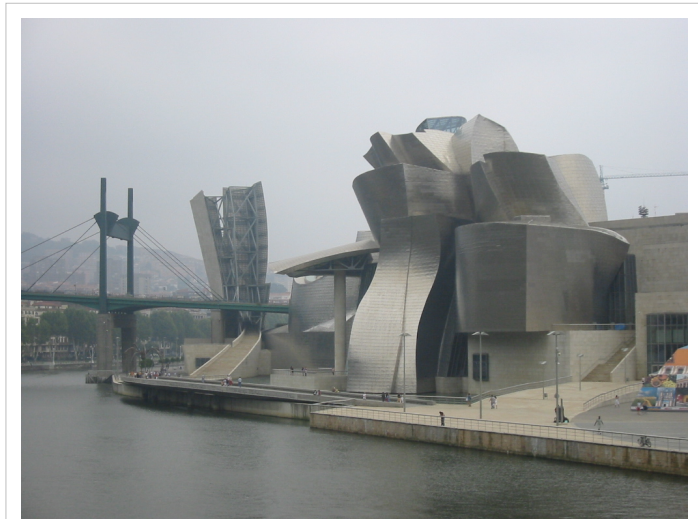
Guggenheim Museum in Bilbao, Spain
