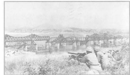
Wrecked bridges over the Han. The Corps of Engineers later rebuilt the Han River bridges.
