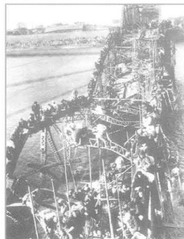
North Koreans fleeing to South over destroyed Taedong River bridge, December 1950.
