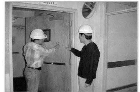
Mr. Wang, Hui-chan (left), HRO Quality Assurance Representative, and Mr. John Ghim, Deputy Resident Engineer, HRO, check the fire door rating on one of the 10 new doors at Yongsan's 121st General Hospital in Seoul.
