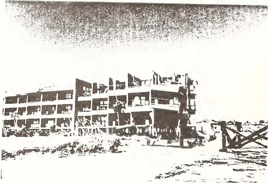
Figure 6. Wind and Surge Damage to Condominium, Isle of Palms.
