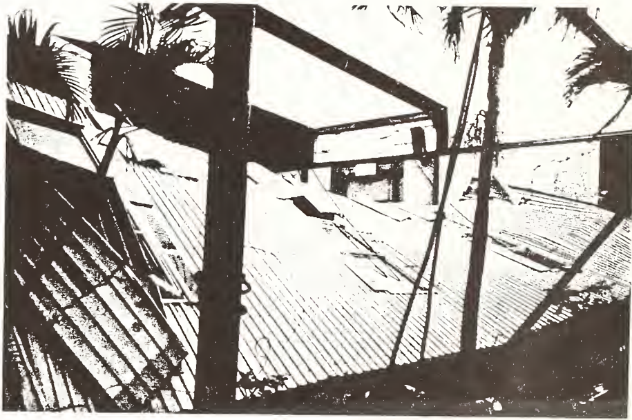
Figure 4. Metal building, Christiansted, St. Croix
