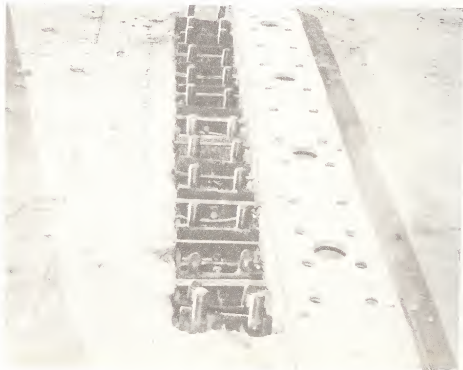
Figure 7 Building 311, Roof level drag-struct shear anchors.
