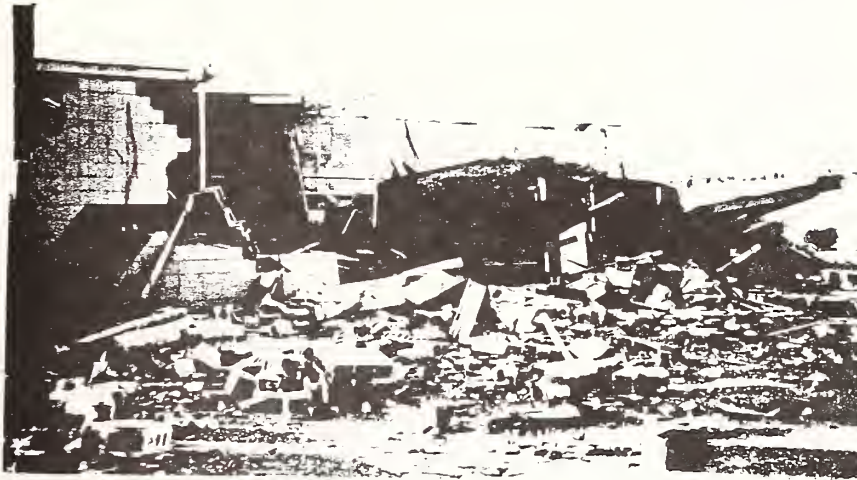
Figure 8. Collapse of Masonry Commercial Structure, Sumter.
