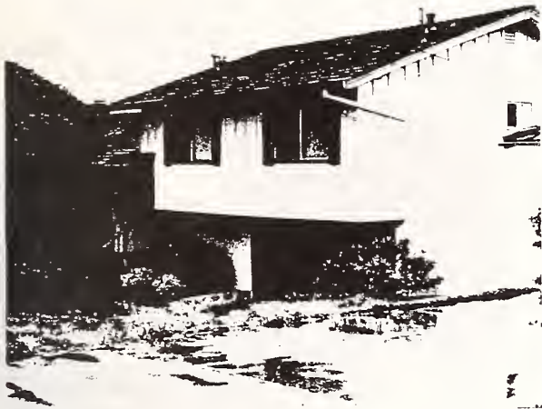
Figure 5. Undamaged split level house located in area of Los Gatos where many older one-story houses slipped laterally off their foundations.
