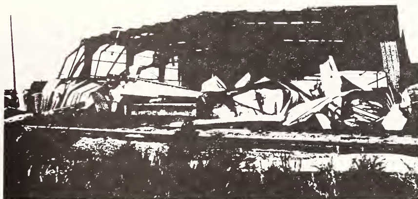
Figure 9. Damage to Metal Building, Charleston.
