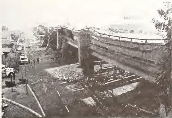
Photo. 2 Collapse of Cypress Viaduct on 32nd Street, Oakland. Typical damage to Type 1 piers (from CALTRANS).
