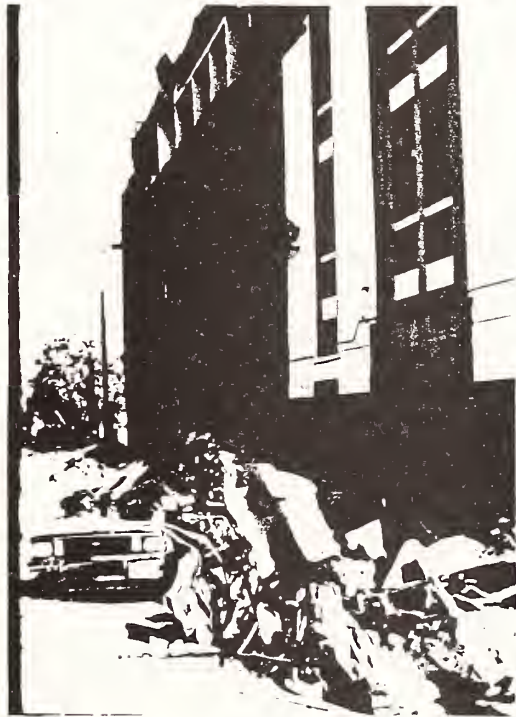
Fig. 4. Cars Crushed by Fallen Masonry, Mission District, San Francisco
