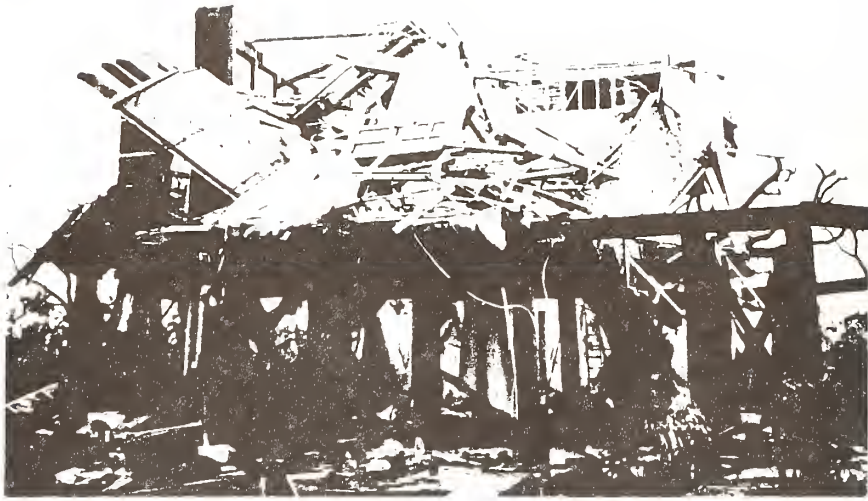
Figure 2. Heavily Damaged House, Bull Bay.
