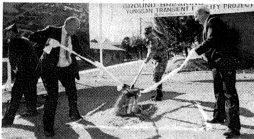
Ed Tohill(L); Chief of Construction and Thayne Coffin(R), Chief of Engineering Division assist Col. Howard Boone, FED Commander, as ground is broken for the Dragon Hill Lodge at Yongsan. There were 3 three-man shovels in use for the occasion (See page 2).
