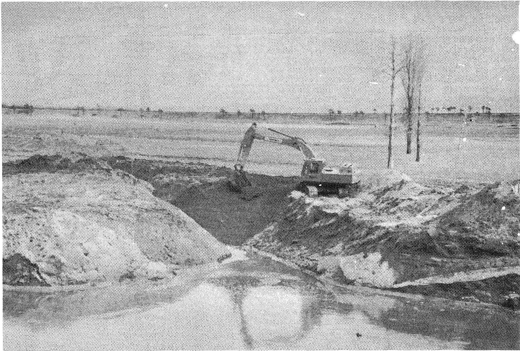
Backhoe fills the excavated area north of the river.
