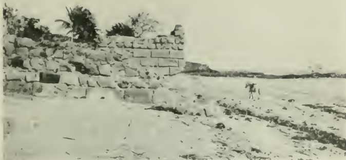
OLD PANAMA, RUINS OF FORT AND SEA-WALL
