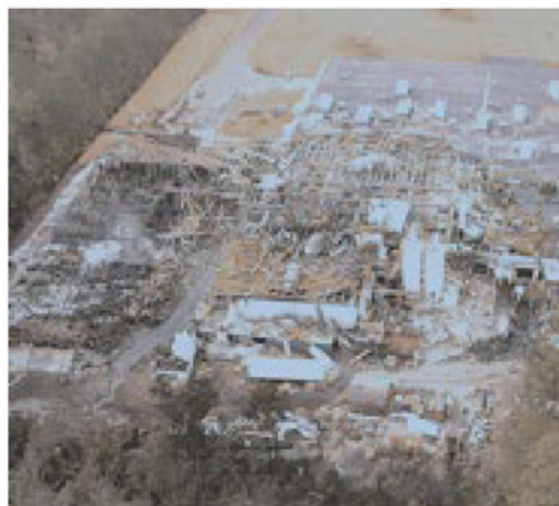
A pharmaceutical plant after a dust explosion.
