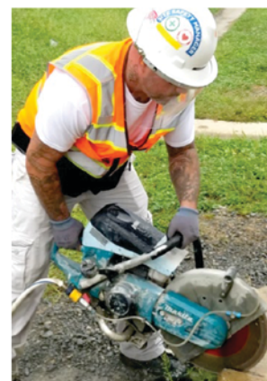
Applying water to the blade of a handheld power saw reduces the amount of dust created when cutting.
