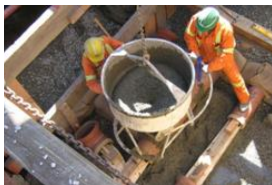
Utility infrastructure maintenance
