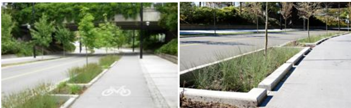
Examples of the sustainable design elements in the Carrall Street Greenway include stormwater infiltration planter boxes, a permeable paver system, and rainwater channels.
