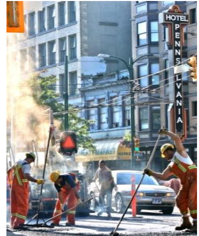
Hastings Street public realm and road improvements
