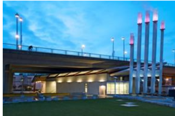
The Southeast False Creek neighbourhood energy utility is an example of a system that uses sewer heat recovery and has reduced carbon pollution by 70 percent.
