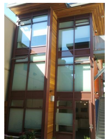
Imouto Housing for Young Women is Canada's first recycled shipping container social housing project
