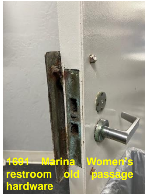
1691 Marina Women's restroom old passage hardware
