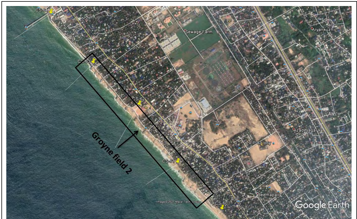
(b) After construction of groyne field 2 (Source: Google earth – 01/2019)
