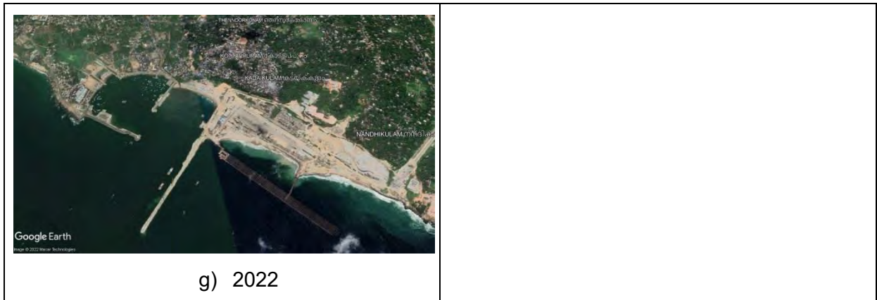
Figure 5-4 Different phases of breakwater construction.
