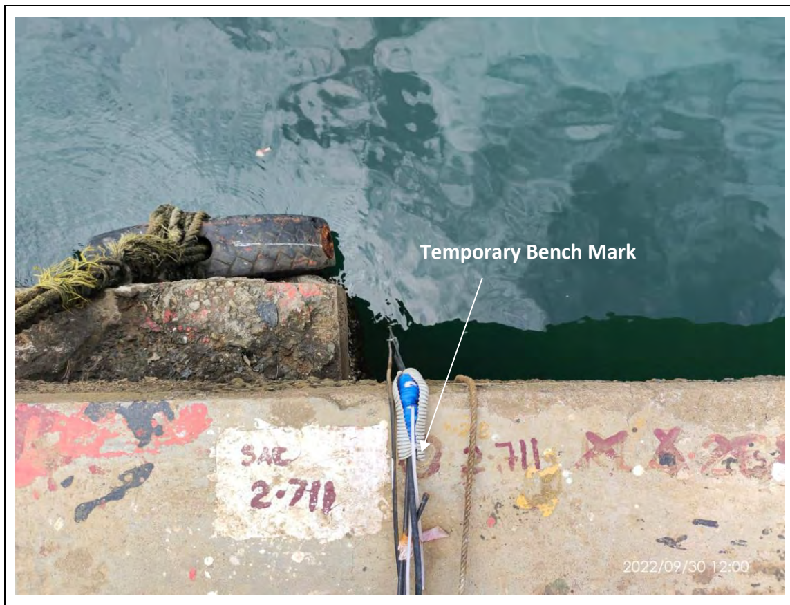
Figure 6-1: Location of TBM
