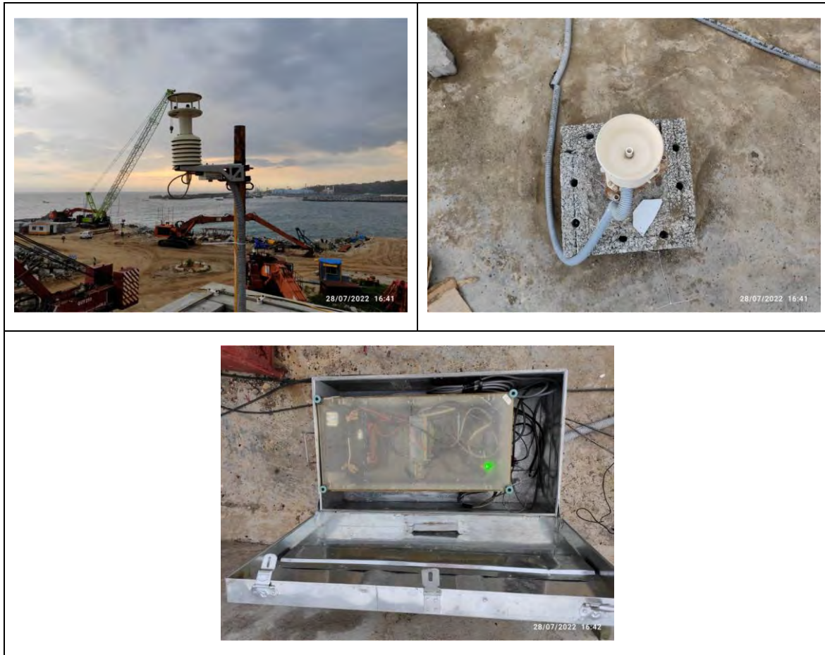
Figure 5-6: AWS on top of Port Control Office building
