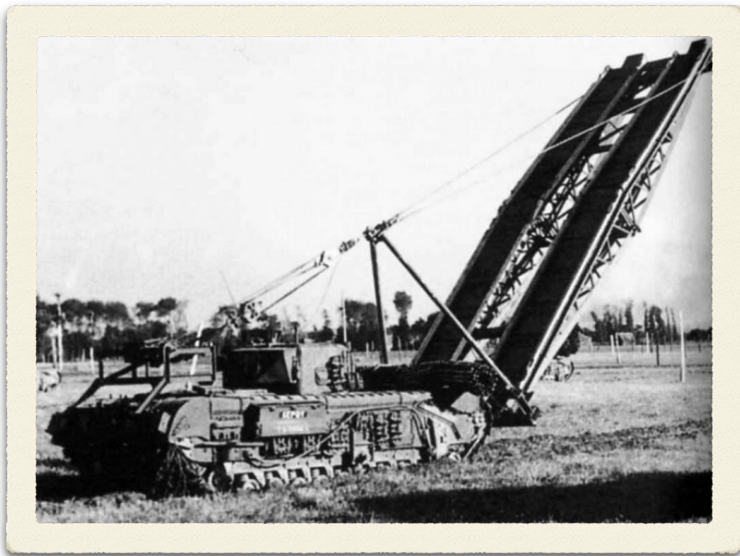
AVRE WITH SMALL BOX GIRDER BRIDGE
