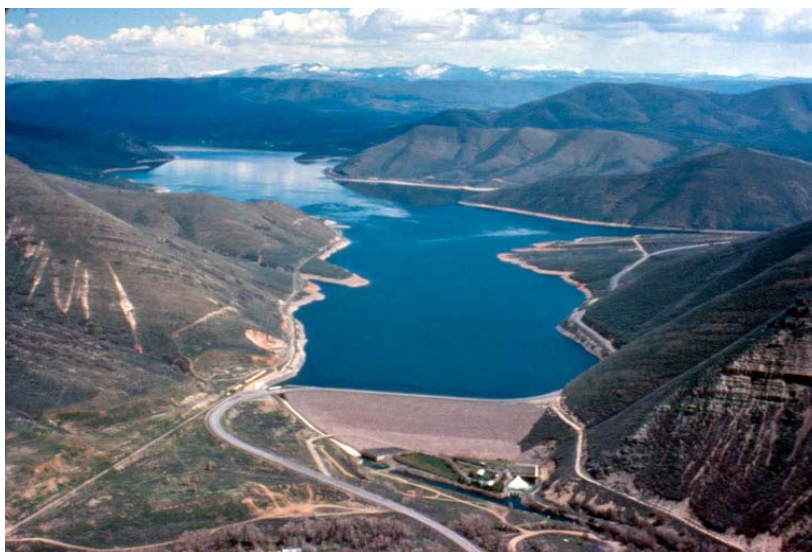
Deer Creek Dam and Reservoir completed in 1941 as part of the Provo River Project, supplying water to many of Utah's residents. (Photo courtesy of Bud Rusho)
