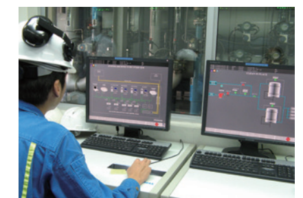
Main control room for field operations
