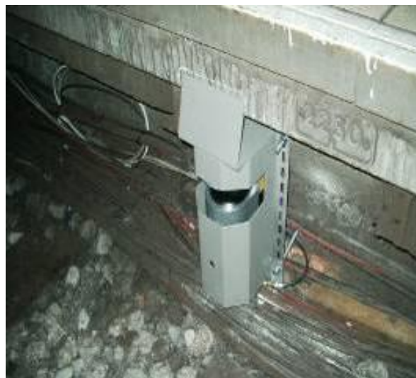
LIDAR scanner on trial at Bank
