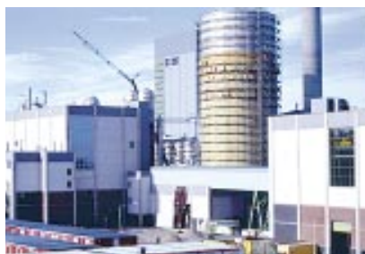
Paroc's biggest delivery of technical insulation in 1995 went to Metsä-Rauma's new pulp mill. More than 10,000 m 3 , i.e. over 100 truckloads, of panel, mat and section insulation were delivered to the plant. Prefabricated insulation segments, a recent innovation at the Lappeenranta plant, made it quicker to insulate the curved pipes.
