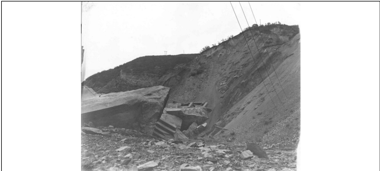
Figure 15. View looking upstream at the base of the left abutment landslide. Note the planar surface of Block 2, which broke along a cold pour joint. The three downed power lines clearly seen entering the slide area in this view had been clipped before the Governor's Board made their site inspection on March 22 nd . Note tandem SCE poles in distance, upstream of the east abutment landslide. Photo by H. Wildey, author's collection.
