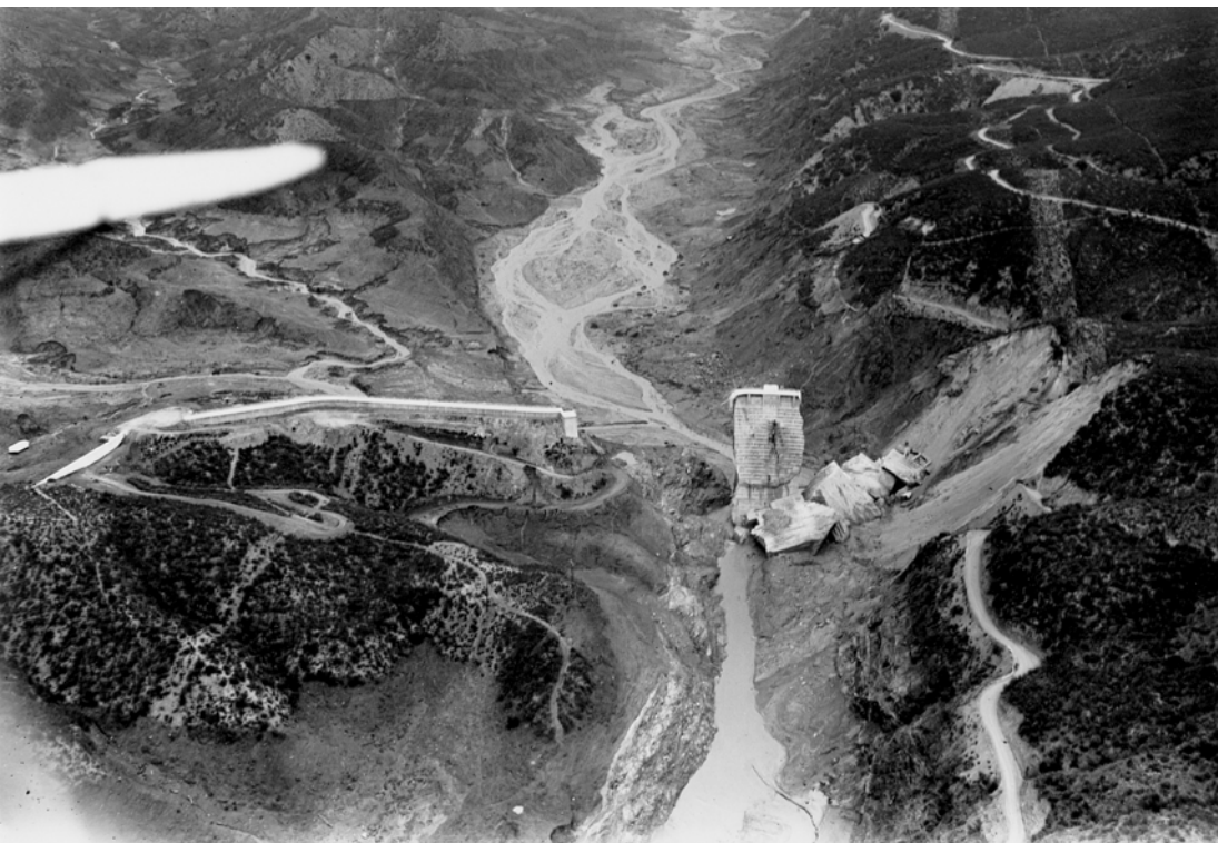
Figure 29. Aerial oblique view looking upstream at the dam area the morning after the failure. Note how high the east abutment landslide extended above the reservoir. Also, note the massive slump block upstream of the dam, caused by rapid drawdown (UCLA Spence Photo Collection).
