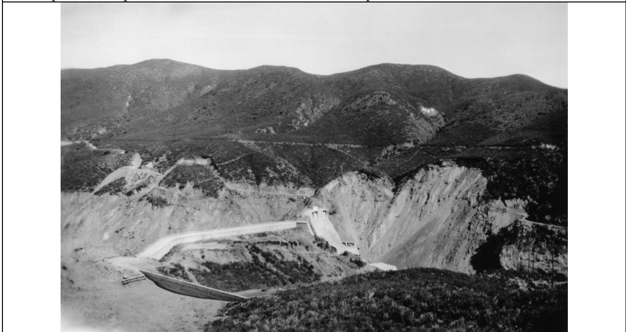
Figure 10 (lower). Same view taken after the failure. Note the prominent topographic bench in the Sierra Pelona escarpment, caused by massive landslipping. The east abutment slide is at right center. Another slump is obvious at left center, which dropped the old San Francisquito Cyn. Rd. about 50 feet (profiled in Fig. 45). From La Rue Collection at the Huntington Library.
