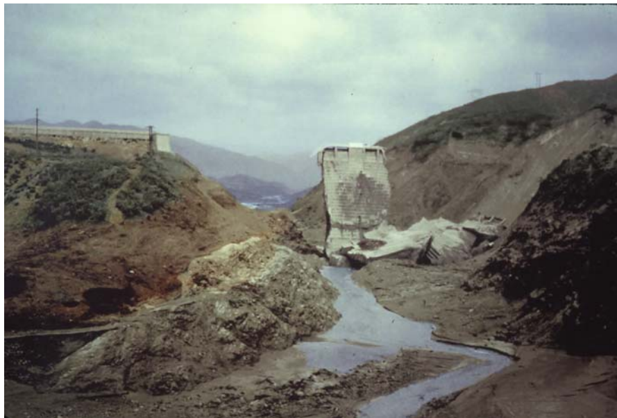
Figure 22. Upstream view of the dam site, taken within five days of the failure, when the downed power lines were still visible, leading into the left abutment landslide. Note position of the intact power poles high above the reservoir water line in background. Photo from C.H. Lee Collection, U.C. Water Resources Center Archives, colorized by Pony Horton.
