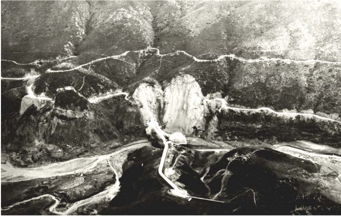
Figure 28. Aerial oblique view of the dam site by Spence Aerial Surveys the morning after the failure. Note the position of the east abutment landslide and old San Francisquito Canyon Road with respect to the dam (from the UCLA Spence Photo Collection).
