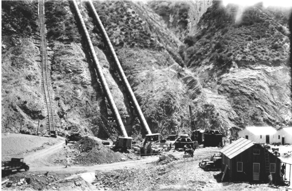
Figure 33. Rebuilding activities at Powerhouse 2 a few weeks after the failure. Surge chamber attendant E. H. Thomas descended the slope along the tramway tracks at left, reaching the high water mark at 12:15 AM, and noting that the flood waters had already dropped 20 feet. The maximum depth of flow here was about 110 feet above the channel (Huber Collection, U.C. Water Resources Center Archives).
