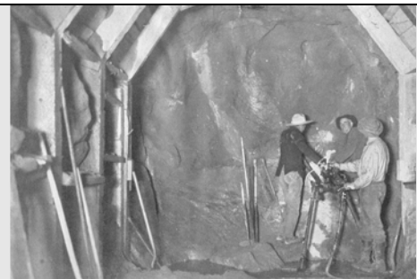
The Elizabeth Lake Tunnel traversed the San Andreas fault at a depth of 400 feet in 1910. Mulholland recognized the threat posed by the fault to the city's aqueduct.
