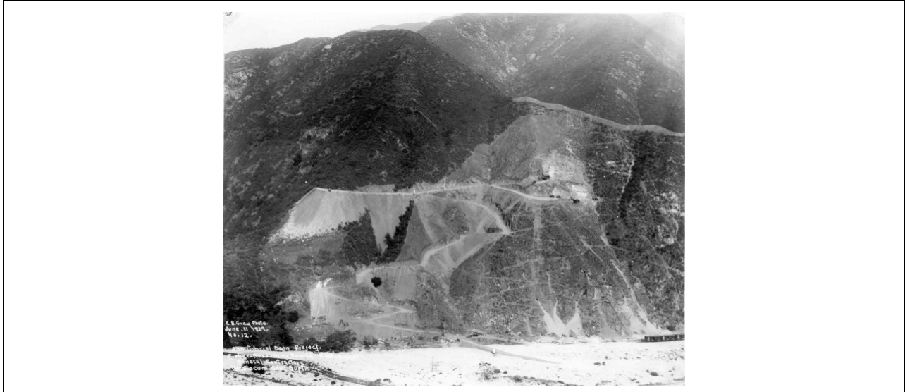
Figure 64. Ten times the size of St. Francis, San Gabriel Dam at The Forks site would have become the largest dam in the world if the State of California had not cancelled the project. This review authority over non-Federal dams by the state was established in the wake of the St. Francis disaster. These images show the excavation activities and landsliding that occurred on the right abutment in 1929. Photos from US Bureau of Reclamation.
