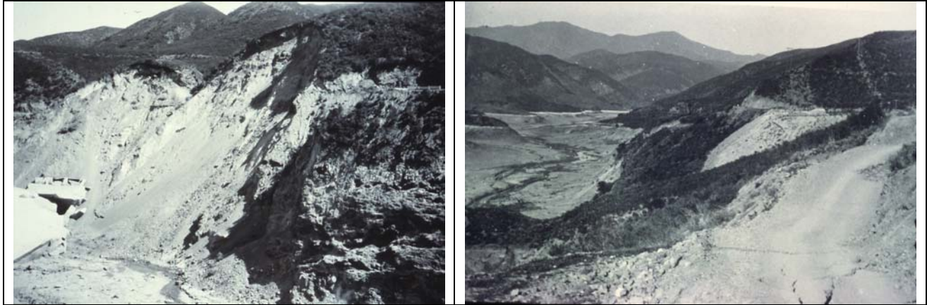
Figure 45. Left photo shows exposed scarp of the east abutment landslide extending well above old San Francisquito Cyn. Rd. Image at right shows gross ground deformations along the Bee Highline Road, about 300 feet above the dam's left abutment. The slope dropped two to nine feet above the east abutment slide. Both photos from Ventura County Museum of History & Art.
