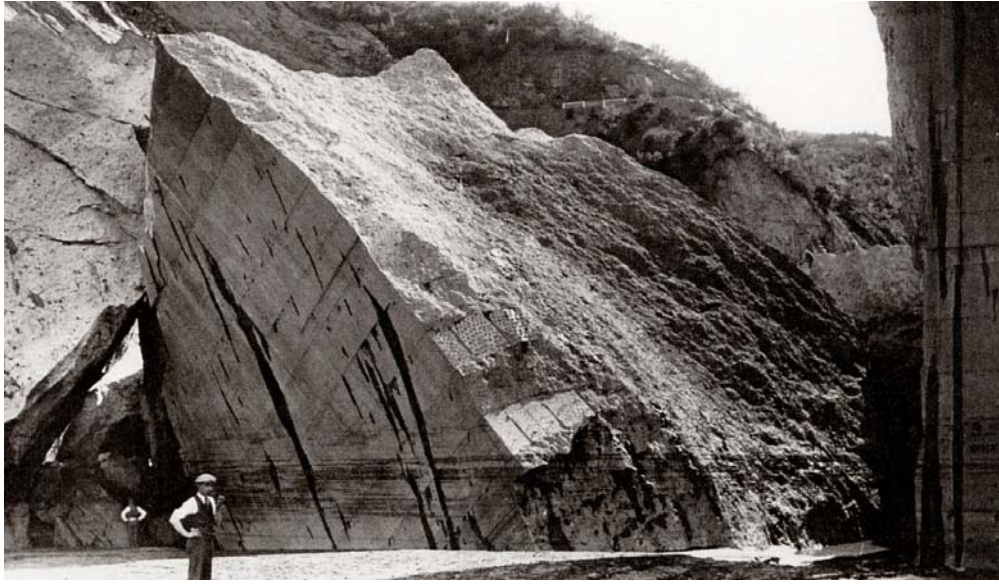
Figure 61. Ground view of Block 2 and a portion of 3, taken after the failure from upstream of Block 1. The horizontal scour marks across the inclined block testify to the reservoir stage when Block 2/3/4 toppled over. The reservoir was only about 17.5 feet deep, or nearly drained, when the left half of the dam's central core fell over. Photo from the W.L. Huber Collection of the U.C. Water Resources Center Archives.
