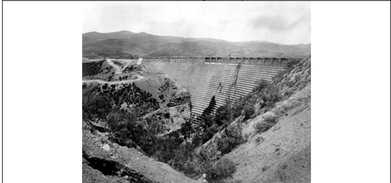
Figure 2 – St. Francis Dam as viewed from the old road, from the left abutment. The old access road with the 18% grade can be seen climbing the right abutment, below the dike. This was where the ‘muddy water’ was observed by damkeeper Harnishfaeger on the morning of the failure. Also note how it would be difficult to notice people with flashlights at the base of the dam’s left abutment, which cannot be seen from the old road.
