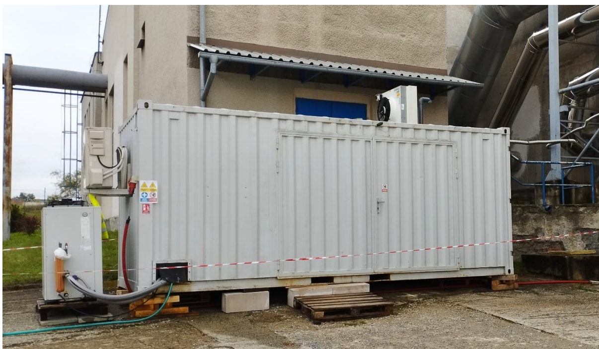
Figure 2. Photo of location of the pilot unit on the ČLT a.s.
