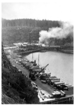
Logging in British Columbia; clearcut, mill, and dock, photograph by H.W. Roozeboom. British Columbia Archives Collection, Royal B.C. Museum Corporation, Victoria (D-05018).
