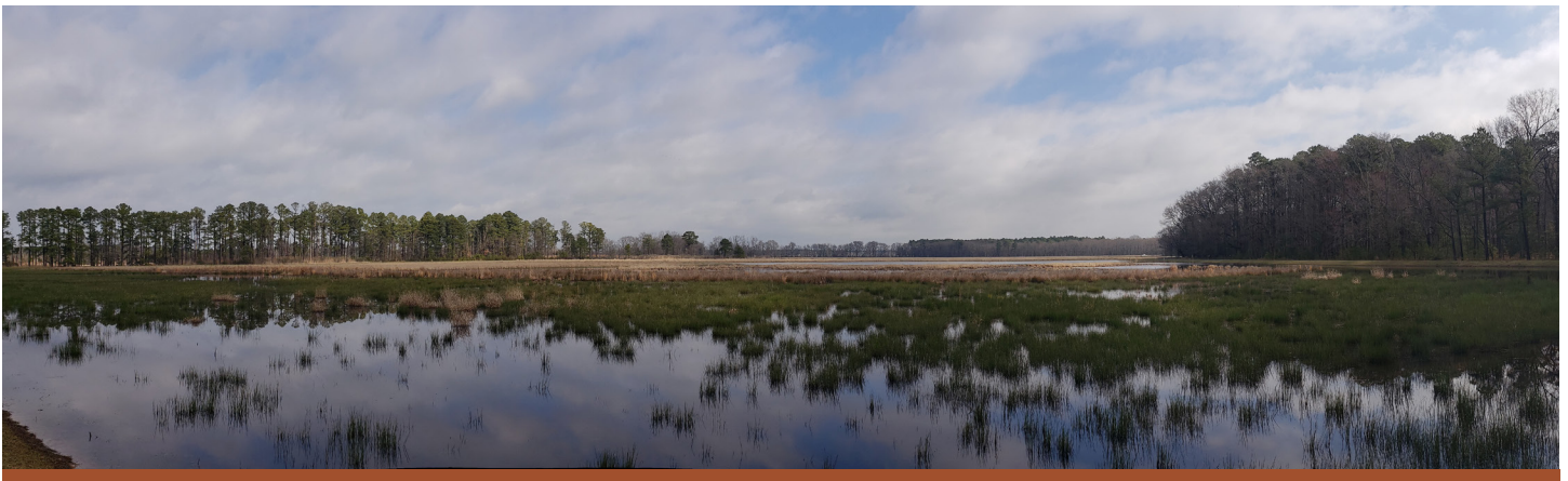
Impoundment at Blackwater six months after construction. Ducks Unlimited
