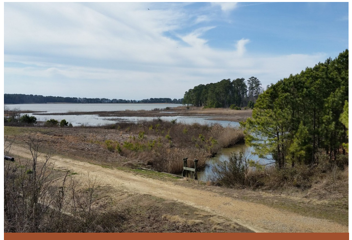
Water control structure on Hog Island, Virginia. New Jersey Audubon Society
