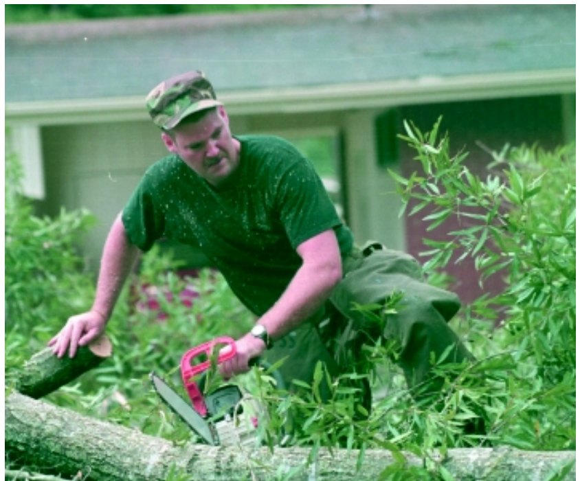
TSgt Lance Filler, 4th CES, removes fallen trees from the Seymour Johnson AFB family housing area. The 4th CES began clean-up immediately after the storm passed. (Photo by SrA Kevin Kuhn)
