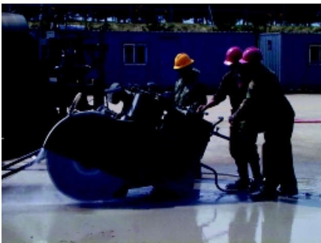
RED HORSE and Air National Guard civil engineers work together to construct an aircraft hangar on a Korean military installation. (Photos courtesy 554th RHS)
