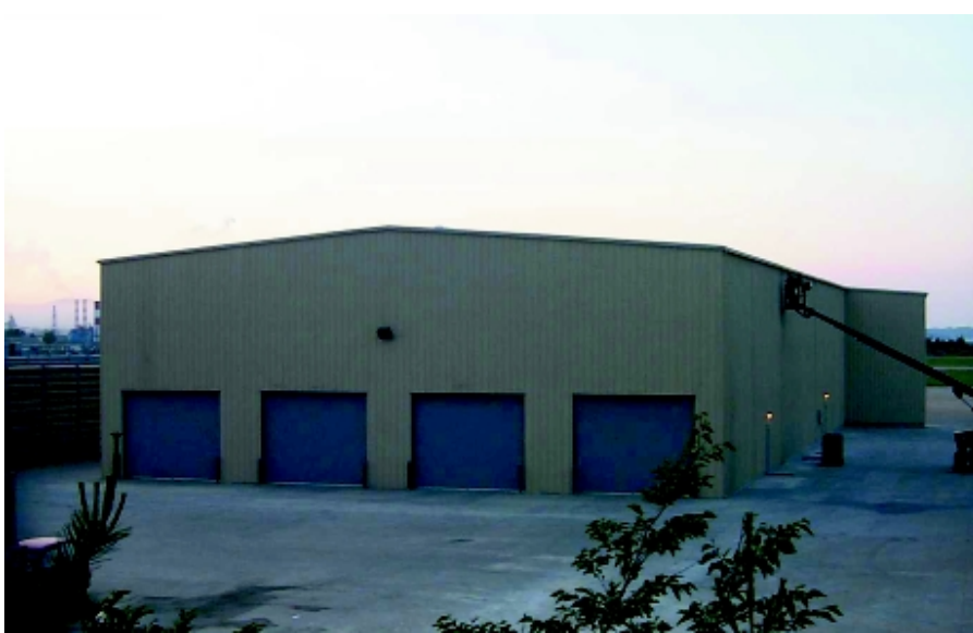
(Top) The front of the 8,000 square foot hangar accommodates an 80 foot by 28 foot hangar door to enable USMC helicopters to be moved into and out of the facility. (Above) The rear of the hangar is for storage of materiel handling equipment with access through four roll-up doors.
