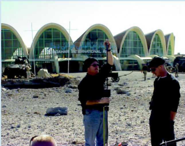
TSgt Steven Russell and TSgt Greg Crosslin conduct pavement tests using a dynamic cone penetrometer at Kandahar International Airport, Afghanistan.
