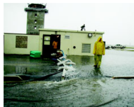
(From top to bottom) Approximately 3 feet of water stood in the basement of Randolph's west airfield vault when the top photo was taken and 4 feet when the second photo was taken. David Washington (in doorway) and SrA Andrew Diehl, both from the 12th CES, at the vault. Approximately 30,000 gallons was pumped out of the basement that day. (Photos by MSgt Luis A. Adams)
