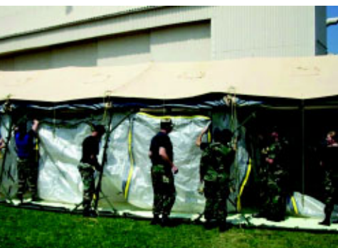
305th CES members practice setting up the new Transportable Collective Protection System, or TCPS. (Photo by Steven Robertson)
