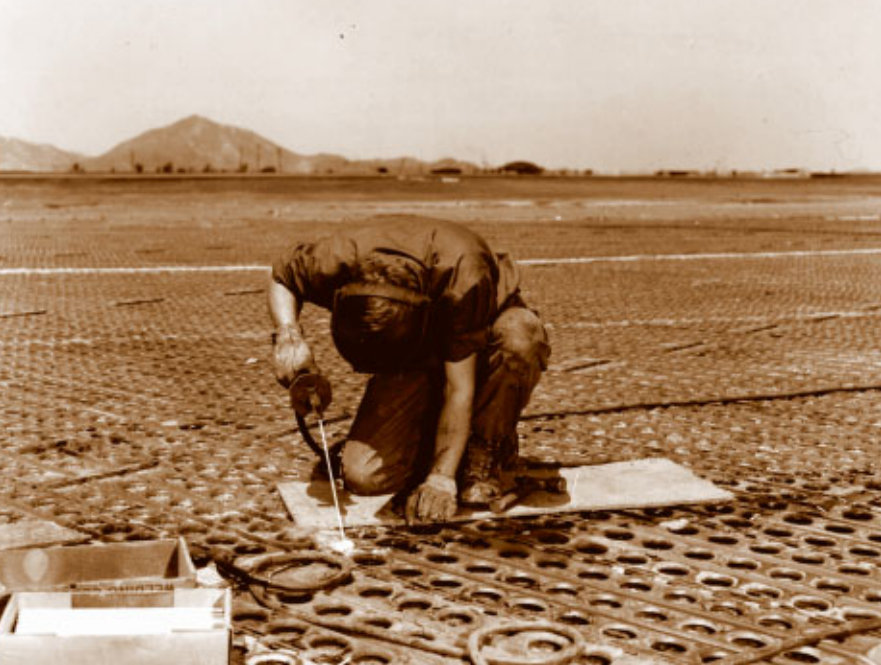
Repair and maintenance of pierced steel planking was a constant job on Korean airfields that saw up to 10,000 takeoffs and landings per month. (All photos USAF unless otherwise noted)
