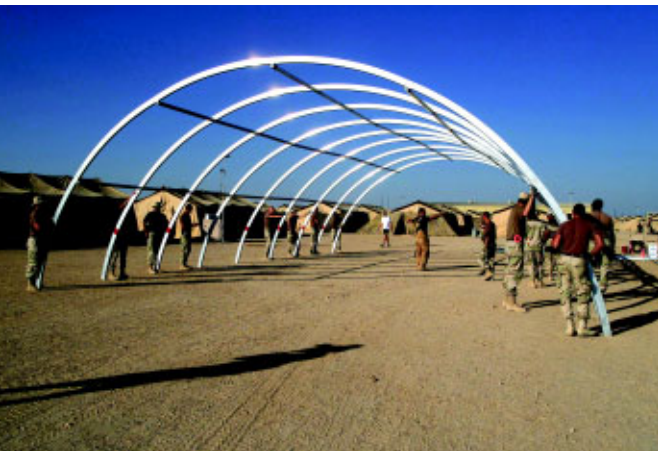
Deployed 552nd CES members erect a California tent during Operation ENDURING FREEDOM, Oct. 30. (Photo by A1C Maryann Walker)
