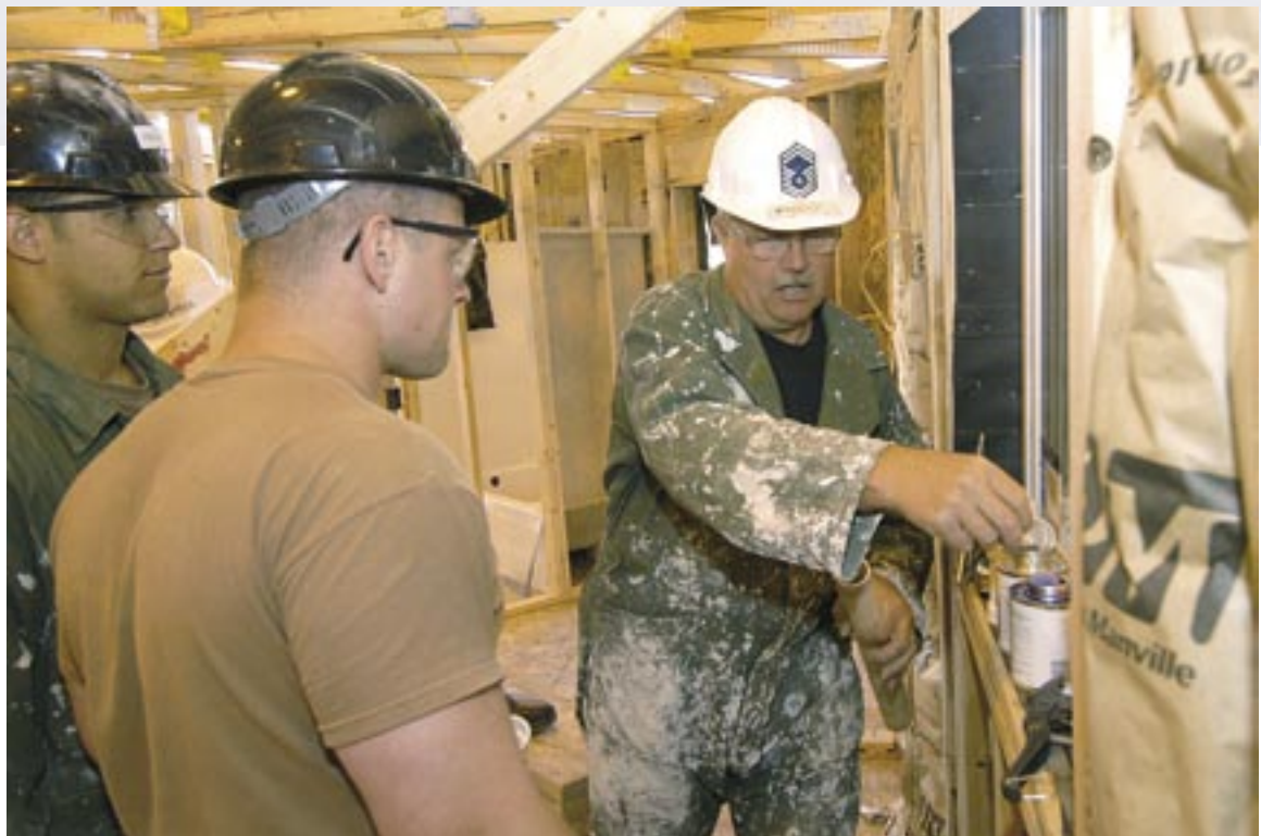
(top) Cadet Monica Wu presents her research poster on groundwater bioremediation. (bottom) SMSgt Gary Kleyn demonstrates the proper technique for priming and gluing PVC pipe to Cadets Kyland Freeman (far left) and Ryan Frost. (photos by Mr. Joel Strayer)
