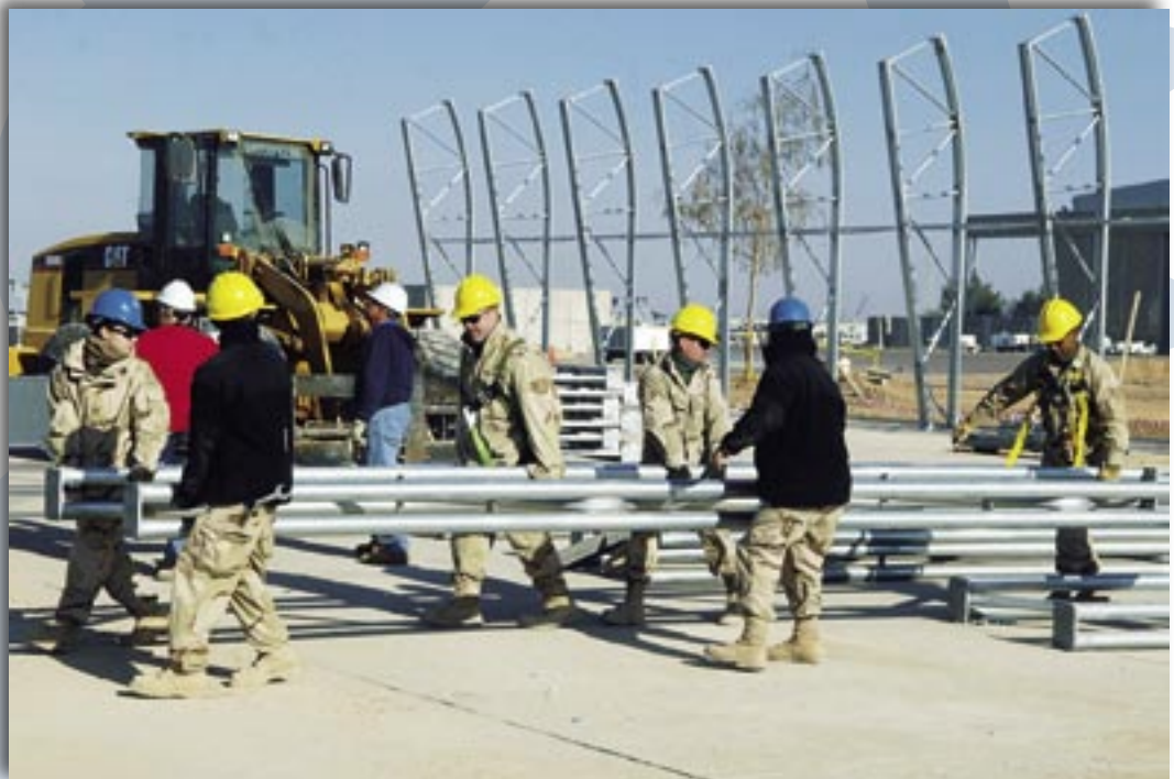
Airmen from the structures shop of the 332nd ECES position an arch during construction of a shelter for Hunter unmanned aerial vehicles at Balad AB, Iraq. (photo by A1C Chad M. Kellum)
