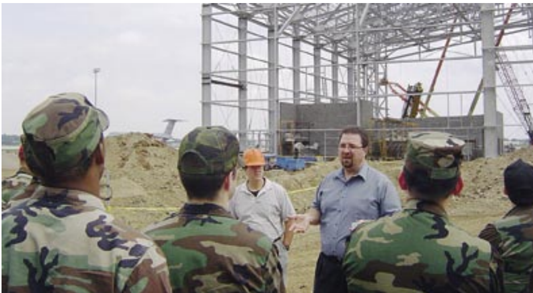
ENG 481 students observe hangar construction techniques as part of their coursework. (photo by Capt Brian Ballweg)
