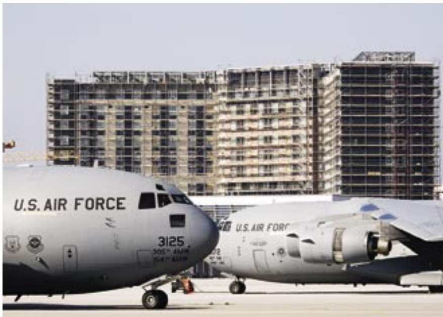
Two C-17 Globemaster IIIs taxi on the busy new ramp while construction of the new hotel continues at Ramstein AB, Germany. (photo by MSgt John E. Lasky)
