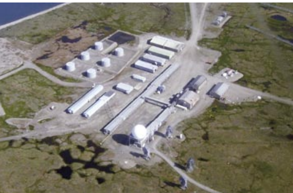
Barter Island Long-Range Radar Site's current configuration is too large for today's needs. (photo courtesy 611th CES)
