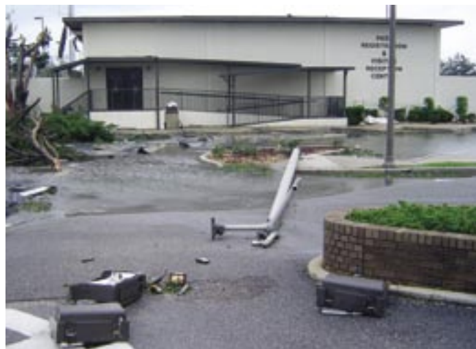
Facilities at Keesler AFB received extensive damage from a direct hit on the base by Hurricane Katrina. (U.S. Air Force photo)
