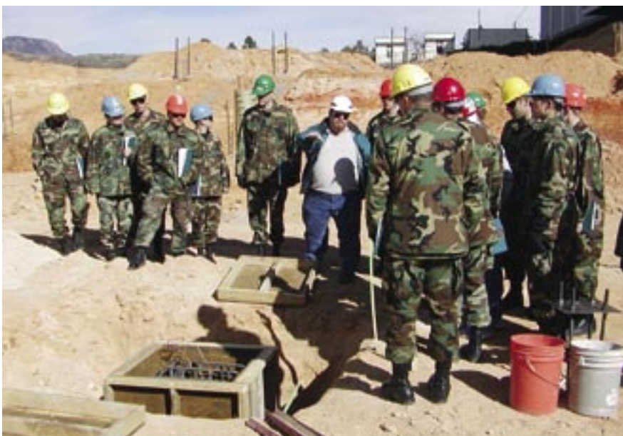
Cadets visit a construction site. (U.S. Air Force photo)
