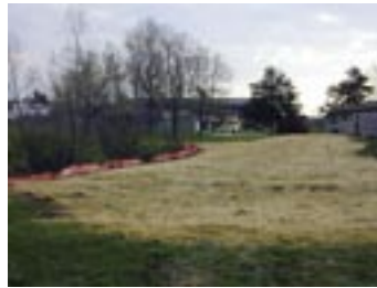
L: Organic mulch and sand from the Base Recycling Center were used to create the biowall at Whiteman AFB. R: After installation, the biowall was hardly noticeable. (photos courtesy CH2M Hill)
