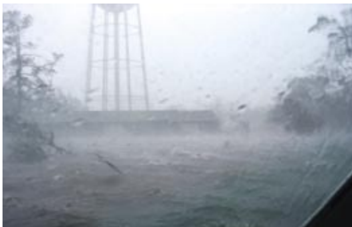
Like the commissary and other facilities, Keesler's thrift store was inundated by the storm surge. (U.S. Air Force photo)
