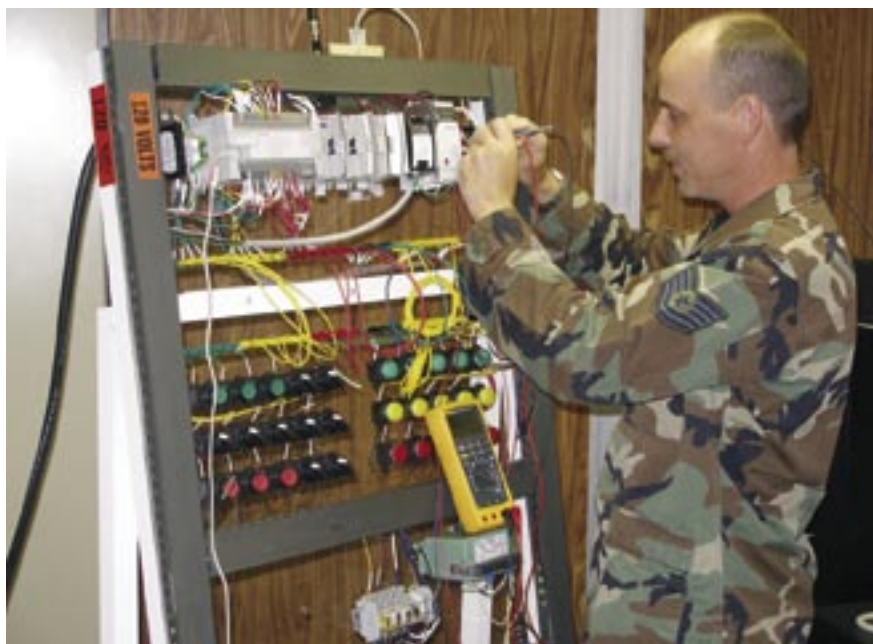
TSgt Christopher Jordan, a SCADA technician, tests the operation of an Allen Bradley Micrologix 1200 PLC destined for installation at Hickam AFB, Hawaii. (photo by author)
