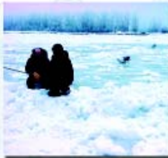
The number of pumps and water source holes depends on how Mother Nature freezes the river. If the ice is flat, as few as four pumps can handle a day's worth of flooding; a "jagged ice" day could involve six pumps, relocated up to three times. (photo courtesy of 354th CES)
