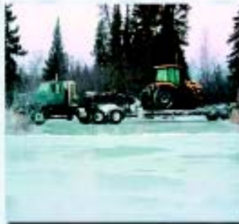
Building up the bridge is a gradual process. With 14" of solid ice, the bridge will support a 4x4 pickup. At 24" you can drive a JD-670 grader over it; at 48", a D-7 dozer. The finished ice bridge can support up to 110 tons. (photo courtesy of 354th CES)
