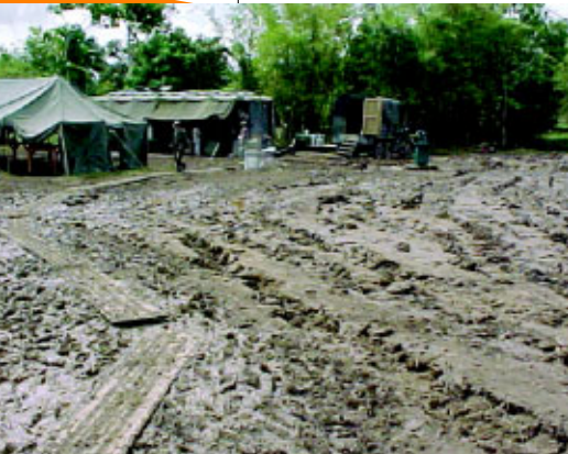
Barely visible in the mud, a metal sidewalk provided some walking access between billeting, dining and shower tents. (Photos courtesy 507th CES)
