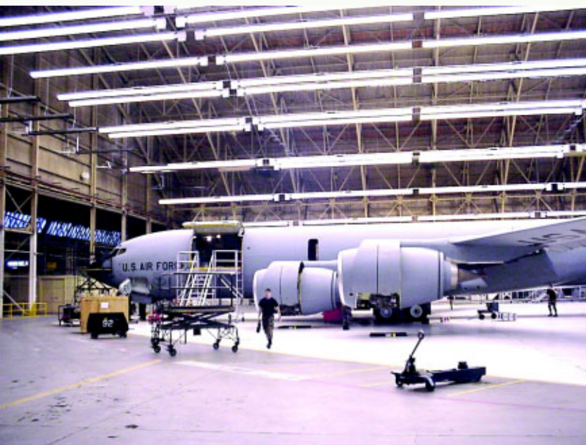
There is literally a “day and night” difference in the new and old lighting systems in the hangars. Photos show Hangar 1 (above) with light pipes installed and Hangar 4 (left) with the old pendant light fixtures. (Photos courtesy 92nd CES)
