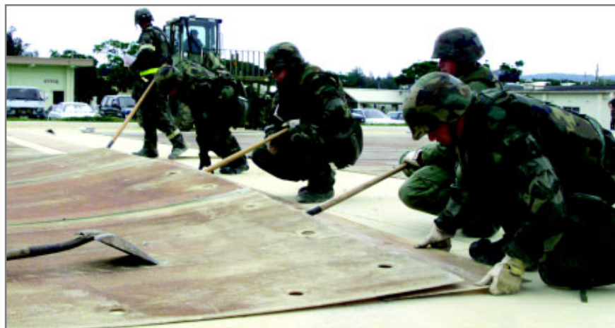
Silver Flag students secure fiberglass matting used to cover holes on the runway. The team, which included three Marines, set a site record for laying down matting the fastest. (USMC photo by Cpl. Denyelle D. Spillane)
