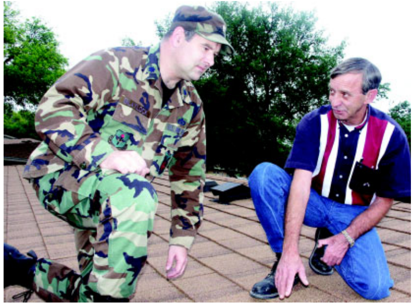
Donald Hendrix discusses a metal roof with Lt Col Michael Blaylock, 47th CES commander, atop a home in base housing. Mr. Hendrix earned an award for his idea to replace asphalt roofs with metal roofs. (Photo by TSgt Anthony Hill)
