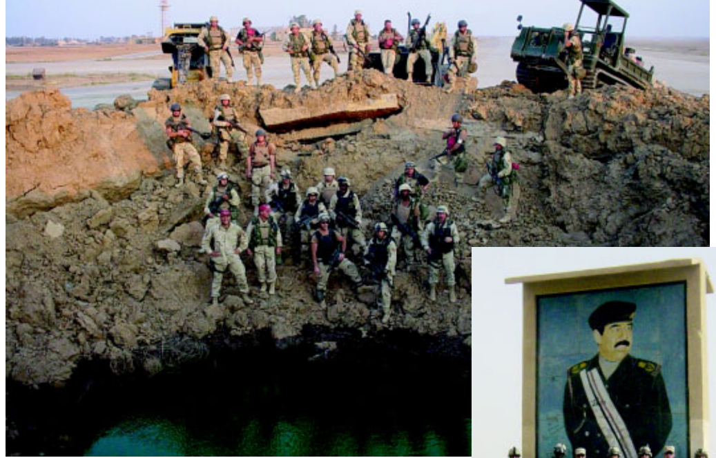
(Above) An Airborne RED HORSE team poses in a crater on a runway at Baghdad International Airport, Iraq, before beginning repairs. The team named it the “mother of all craters” as it was 135 feet wide, 40 feet deep and filled with water 15 feet deep. Brig Gen Pat Burns, the Air Combat Command Civil Engineer, said the crater was well over twice the size of any crater repaired in training or combat. RED HORSE is repairing the civilian and military runways at Baghdad IAP, a primary base of operations for U.S. troops, cargo and humanitarian airlift for Operation IRAQI FREEDOM. (Right) ARH members pose in front of a portrait of Saddam Hussein near Tallil AB. (Photos courtesy HQ ACC/CEX)
