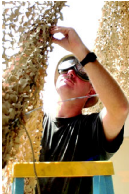
SSgt Virgil Deaton, 320th ECES, uses zip ties to join two pieces of camouflage netting together. Sergeant Deaton was covering the "Sun Screen" his shop built and set up over the CAT Scan Complex near the 320th Expeditionary Medical Squadron.
