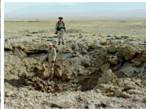
(Left) MSgt Ron Westerfield measures a typical spall in front of one of the craters on the runway during the team's initial evaluation in November. (Above) MSgt David Cook (in crater) and MSgt Westerfield examine a typical runway crater. (Photos courtesy 823rd RHS)
