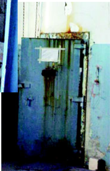
No appreciable real property maintenance had been performed inside Hangar 5 for more than 25 years, leaving it unfit for aircraft maintenance and in very poor condition. Photos show eroded doorframe and wall damage inside Hangar 5.
