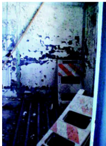
No appreciable real property maintenance had been performed inside Hangar 5 for more than 25 years, leaving it unfit for aircraft maintenance and in very poor condition. Photos show eroded doorframe and wall damage inside Hangar 5.
