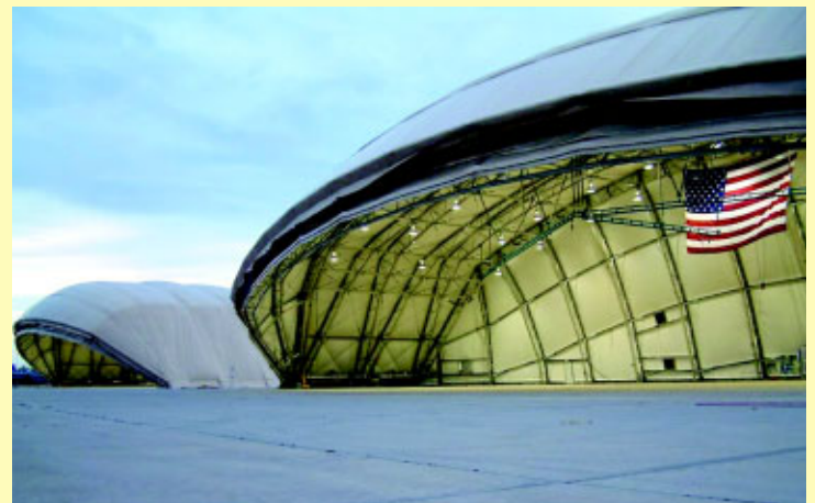
Members of the 49th MMS erected two portable shelters for B-2s at a deployed location. (Photos courtesy 49th MMS)
