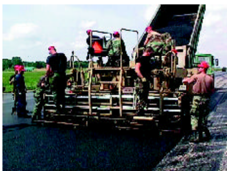
Airfields Flight members pave Taxiway Echo at Taszar, Hungary.
