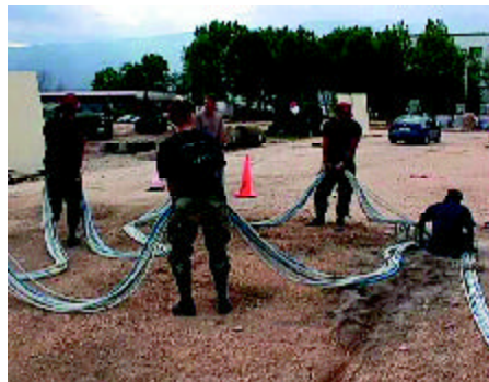
Installing primary distribution cable at Aviano AB, Italy.
