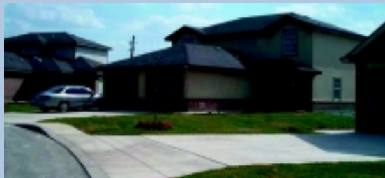
More than 420 new homes for enlisted service members E-3 to E-7 are nearing completion at Lackland AFB. This was DoD's first housing privatization project. (DoD photo by Linda Kozaryn)
