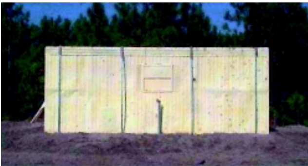
Blast test results on a 10-foot by 20-foot construction trailer with a polymer retrofit applied to both the inside and outside. With only minor structural damage occurring to the trailer, the interior space was completely survivable.
