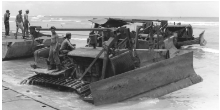
The 1884th and 1887th Engineer Aviation Battalions build a protected harbor at Saipan Village on Angaur Island in the Caroline Group. Here, giant bulldozers pull pontoon causeway to a new position, Oct. 1944.
