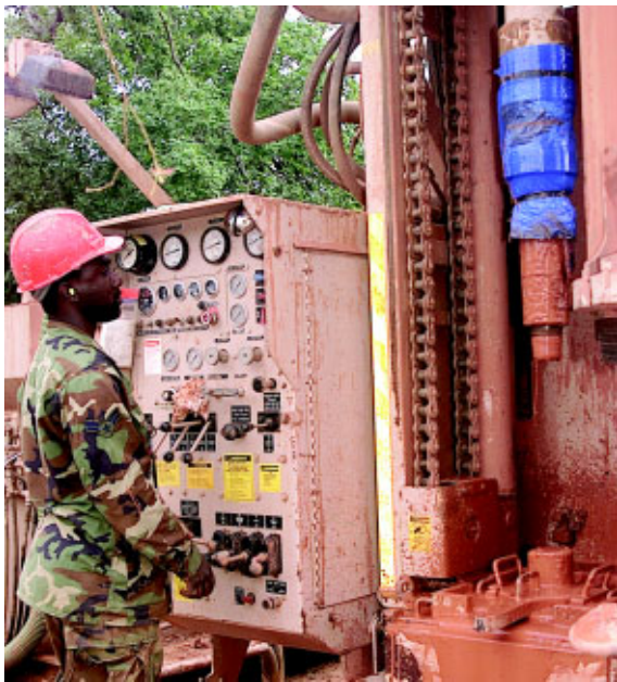
A1C Romeo Peart, 823rd RHS, pulls the drilling steel from the water well drilling machine at Estigarribia, Paraguay. (Photo by SSgt Richard Freeland)
