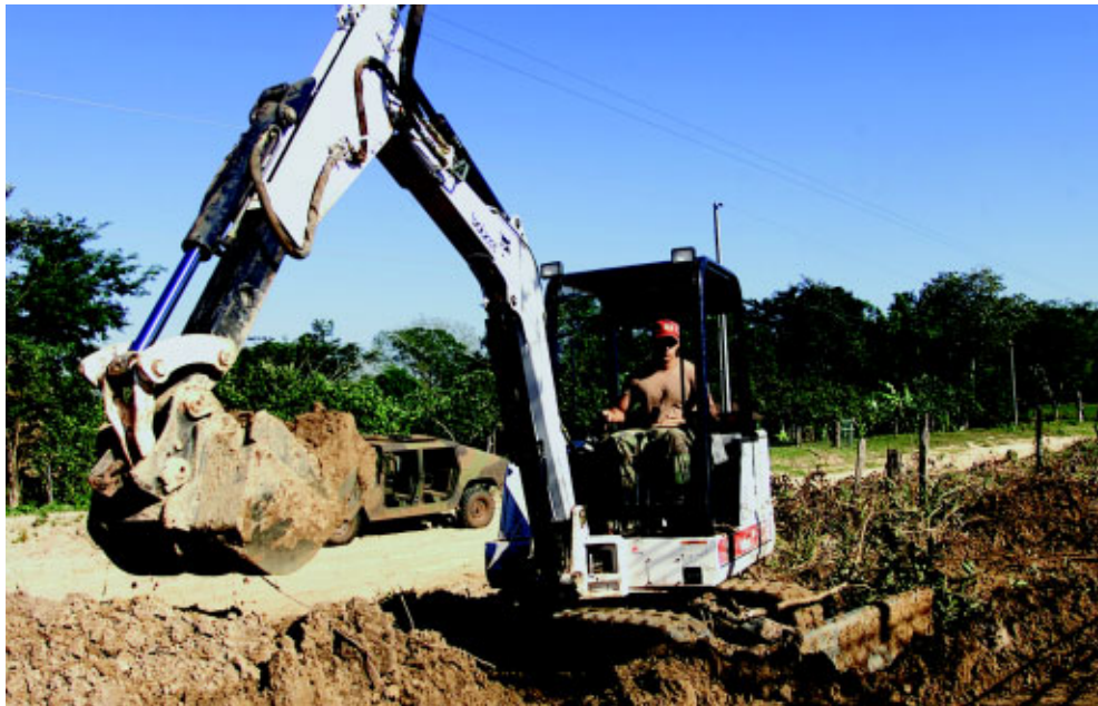
SSgt Bryan Manchester, 823rd RHS, uses a bobcat with excavator to fill the well tower base with dirt after securing it with cement during construction of a well at Las Palmas, Paraguay, in May. (Photo by SSgt Maritza Fernandez)
