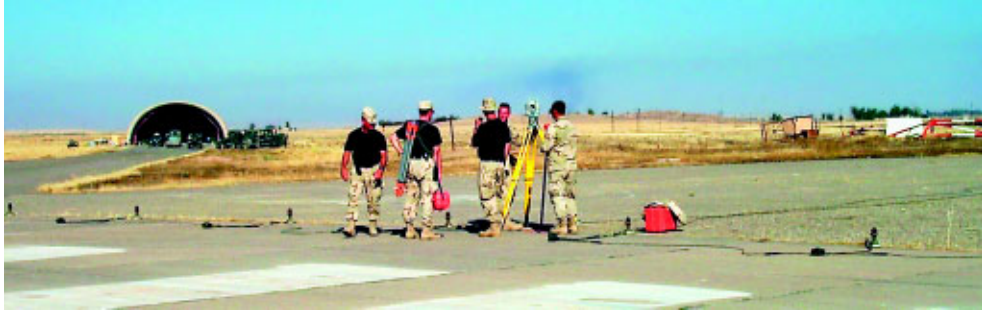
CEMIRT technicians and 506 AEG/ECES engineers survey to pinpoint visual navigation aid locations at Kirkuk AB, Iraq.
