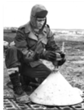
On the cover: An Air Force civil engineer performs maintenance on runway lights in Korea during the winter. The runway is made of pierced steel plank. (U.S. Air Force photo)
