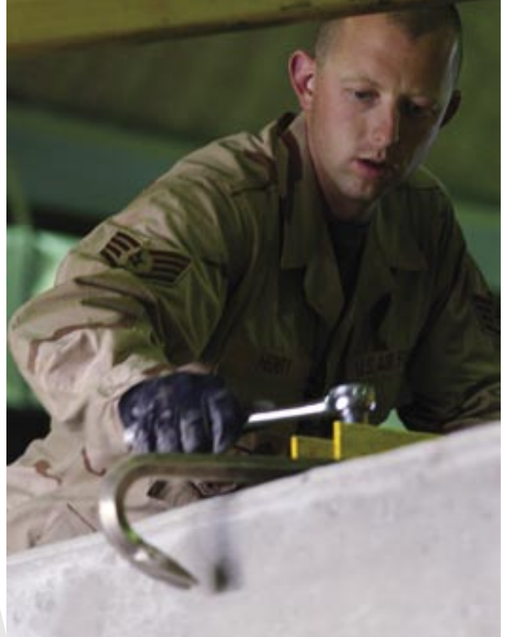
SSgt Justin Henry, 332nd ECES, attaches 10-foot metal arms to a concrete block for placement at an entry control point at Balad AB, Iraq. (photo by TSgt Jennifer Gregoire)
