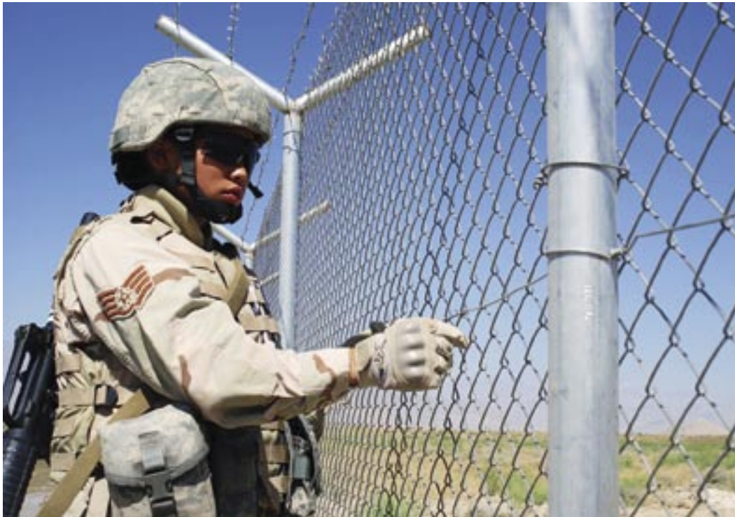
SSgt Rebecca Cook, 755th ECES engineering technician from Eglin AFB, Fla., and expansion project manager, performs a fence tie inspection at the expansion project. (photo by the author)
