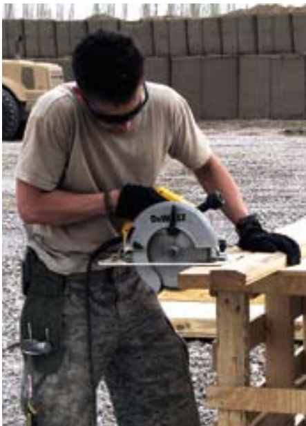
(Left) A1C John Owings saws wall studs at the new Joint Combat Outpost Milledge, Iraq. (photo by A1C Nicholas Lane) (Right) SrA Dan Smith, SrA Dion Williams, A1C George Farrington, and A1C Richard Simmons pour and rake concrete pads at FOB Caldwell, Iraq. (photo by SSgt Josh Jeffreys)
