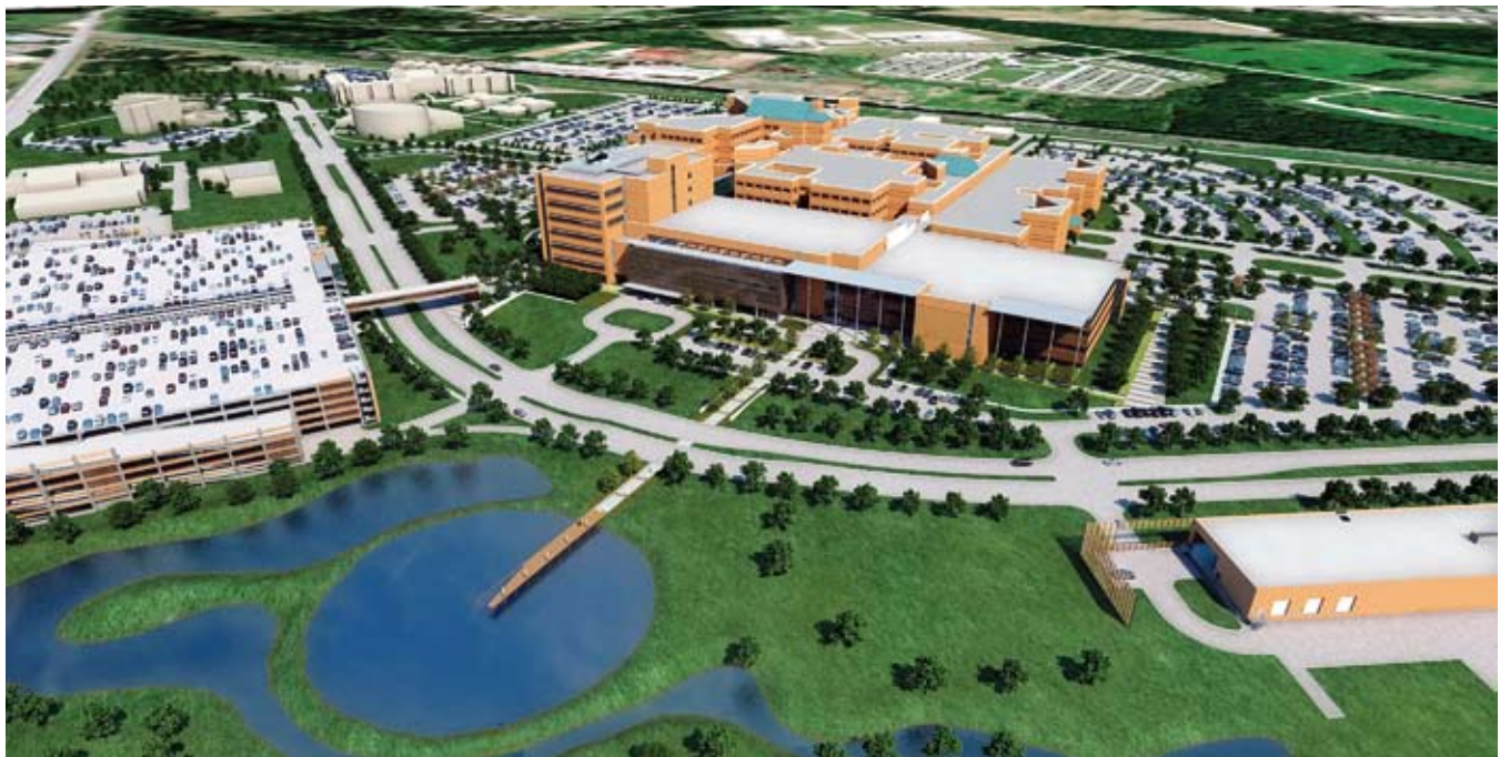
An aerial view rendering of SAMMC-North showing the 760,000 square foot addition (center) that covers the entire front of the existing Brooke Army Medical Center. (Approximately 288,000 square feet of the existing BAMC facilities will be renovated.) A 5,000 space parking garage will also be built (far left in middle), as well as a central energy plant (lower right corner). (Graphic courtesy of the U.S. Army Corps of Engineers)
