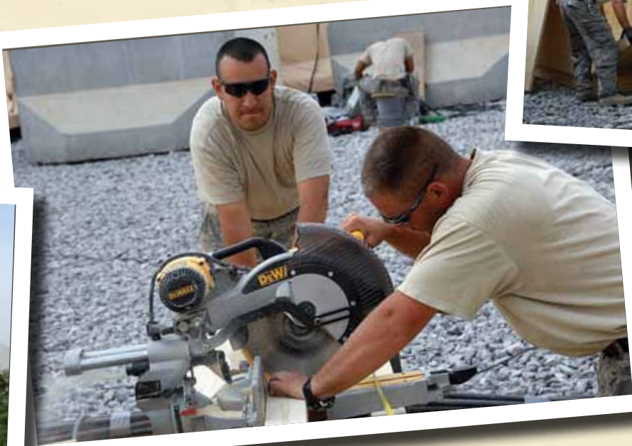
Photo left: A member of the 777 EPBS records GPS coordinates while surveying a location near Kandahar. (U.S. Air Force photo); Photo center: At Access Control Station 2, Kandahar City, Afghanistan, SSgt Joel Carrerra, left, and TSgt Mathew Bashaw, both utilities technicians assigned to the 777 EPBS cut trusses for a medical aid station. Photo right: 777 EPBS Airmen build a medical aid station. (photos by MSgt Samuel V. Ameen)
